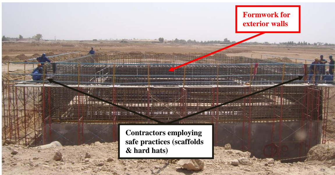
Site Photo 14. Effluent pump station construction
