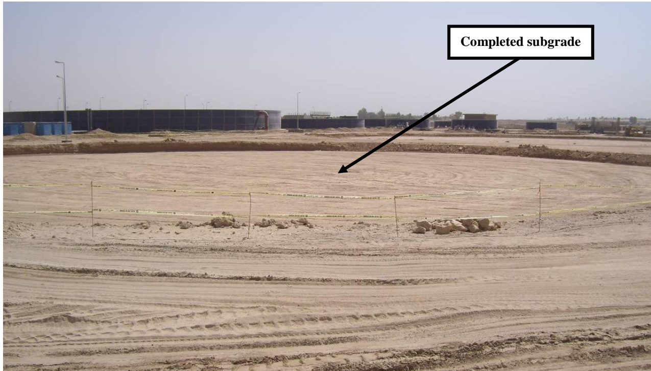
Site Photo 7. Aeration tank subgrade
