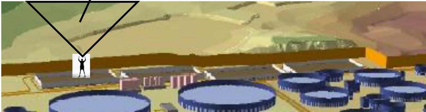
Figure 7. Portion of the WWTP (sludge drying bed area)
