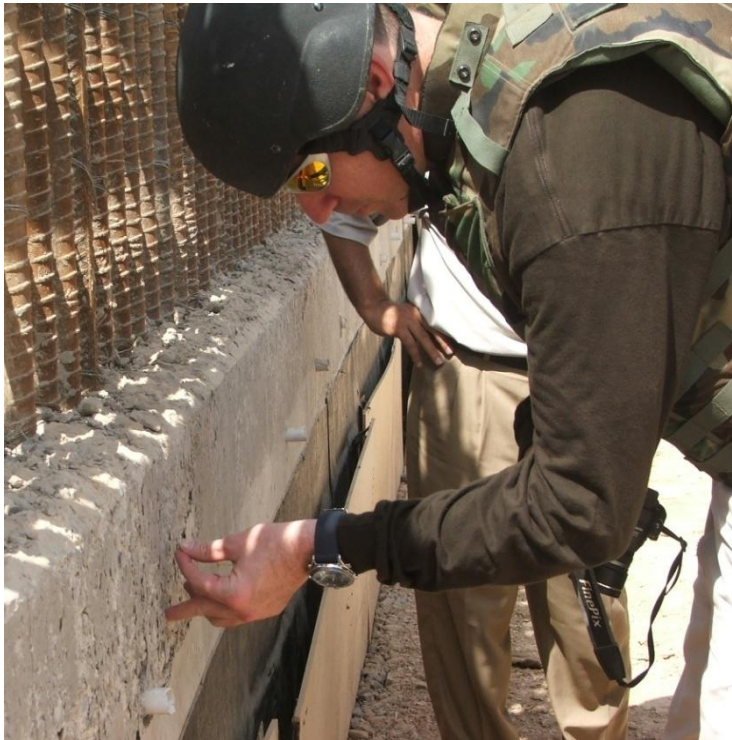
Site Photo 20. SIGIR Inspector checking concrete work
