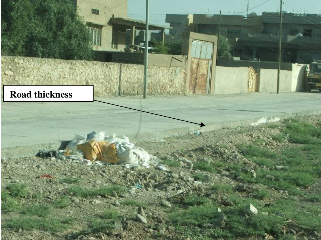
Site Photo 9. Newly constructed road thickness
