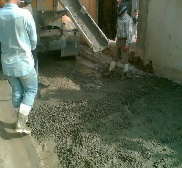
Site Photos 4 and 5. Concrete pour and newly constructed road leveling (Photo courtesy of USACE)
