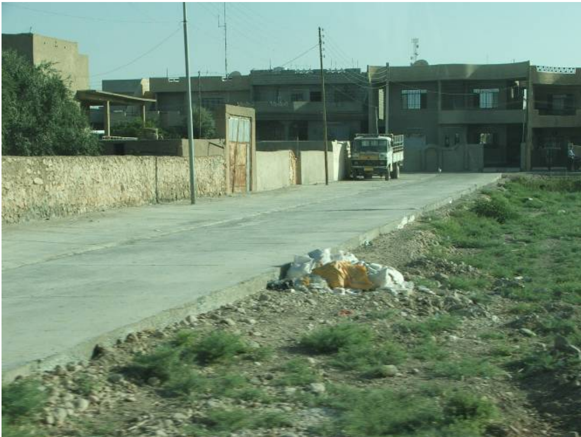
Site Photo 8. Newly constructed road cleared of debris.
