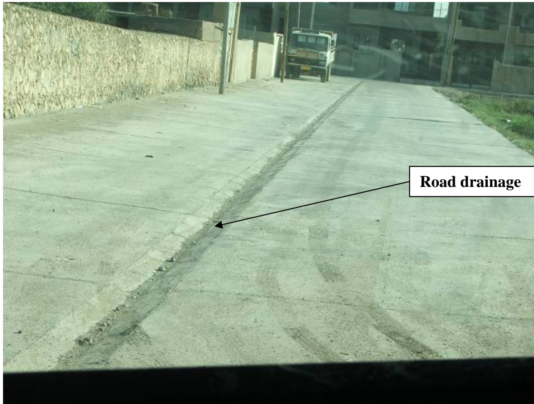
Site Photo 10. Newly constructed road drainage
