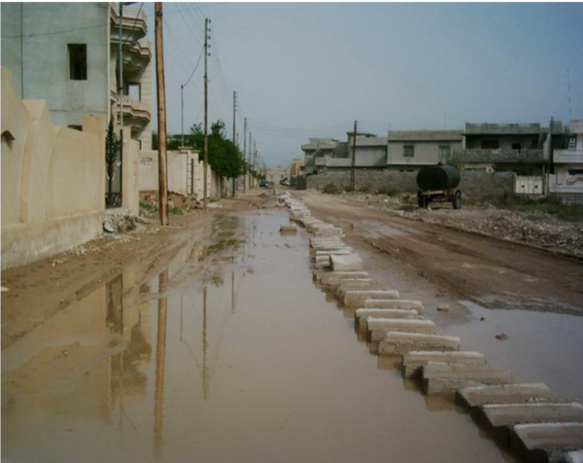
Site Photo 1. Condition of road prior to construction (Photo courtesy of USACE)
