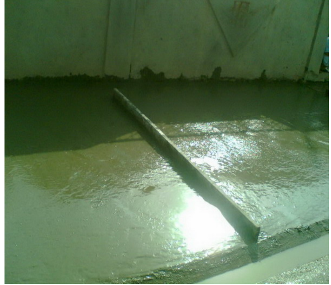
Site Photos 4 and 5. Concrete pour and newly constructed road leveling (Photo courtesy of USACE)
