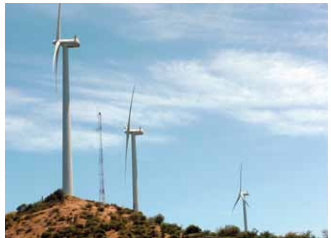
NAVAL STATION GUANTANAMO BAY, CUBA (Mar. 29, 2005) At 80 meters (262 feet) high, the three-blade wind turbines are among the most noticeable features at Naval Station Guantanamo Bay, Cuba. (U.S. Navy photo by Kathleen T. Rhem)
