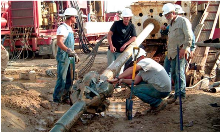
HDD rig with backreamer.
