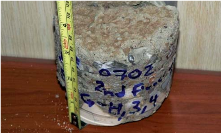
Measurement of a concrete core sample that did not meet contract specifications. (USACE photo)
