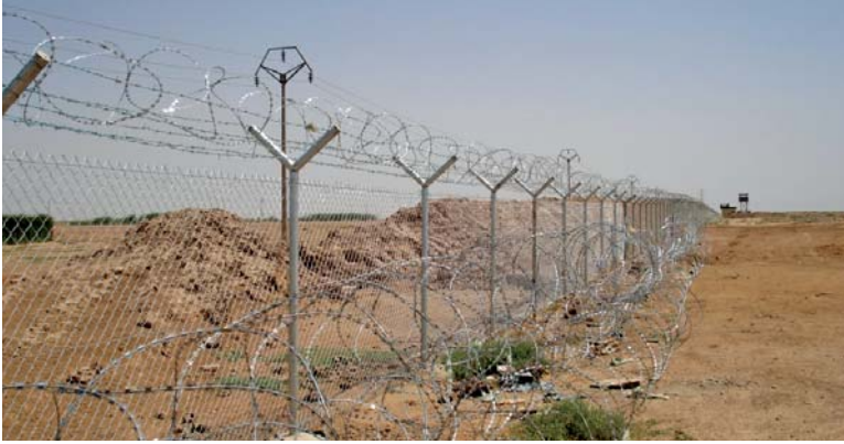
Chain-link fence and barbed wire along Phase 3 of the pipeline exclusion zone for the Kirkuk-to-Baiji pipeline.
