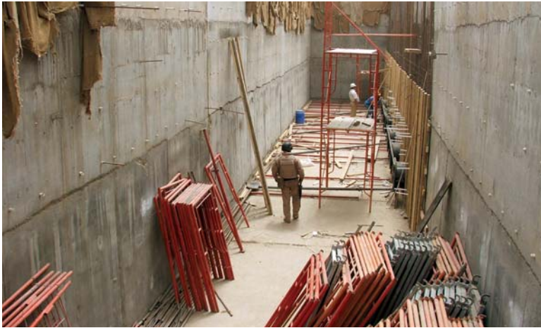
Pump station under construction at the Falluja Waste Water Treatment Plant.
