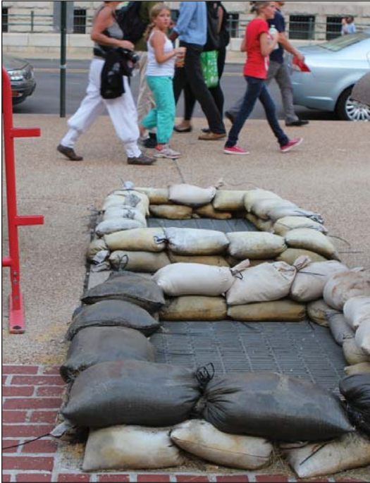
▲ Using sandbags is a short-term, economical solution but does not reduce flooding.
