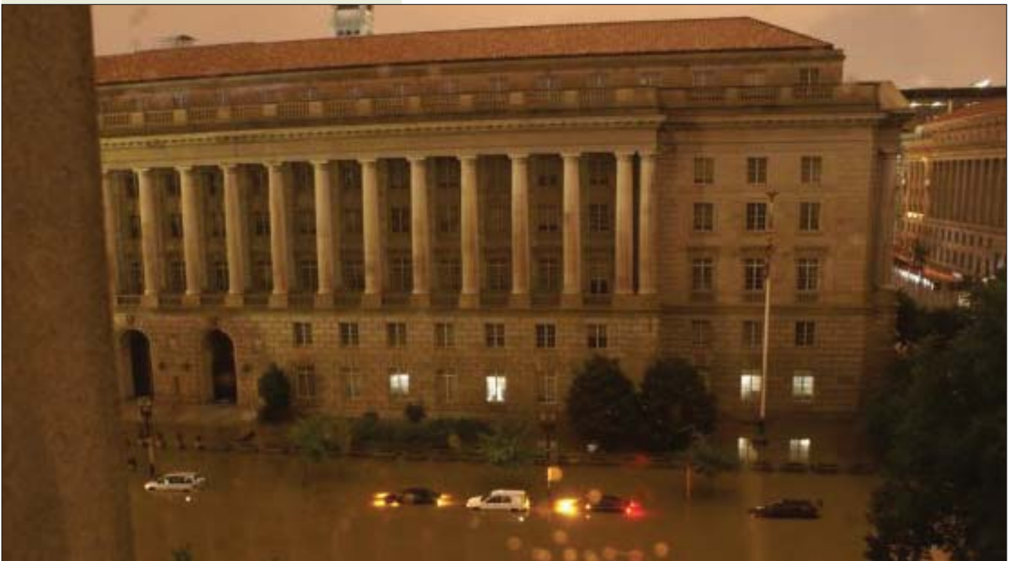
▲ Stormwater flooding after a designated 200 year storm event; June 2006.
