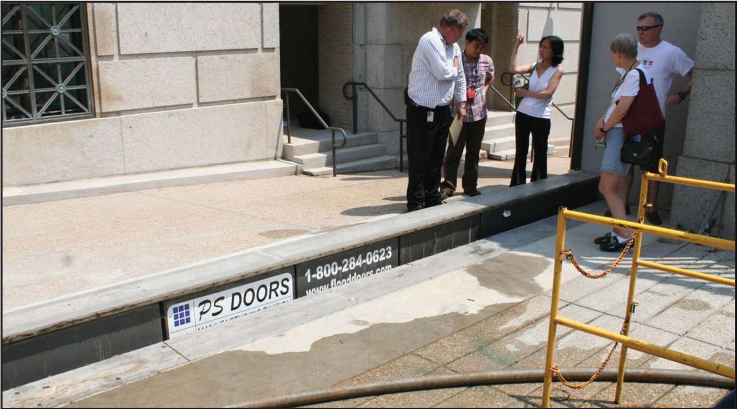
▲ Since the 2006 flood, the National Archives has installed floodproofing elements including self-rising flood gates and watertight doors.
