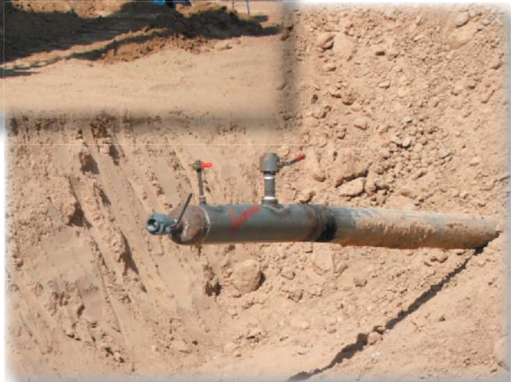
Pipe with hydro-test fittings at river crossing in northern Iraq.
