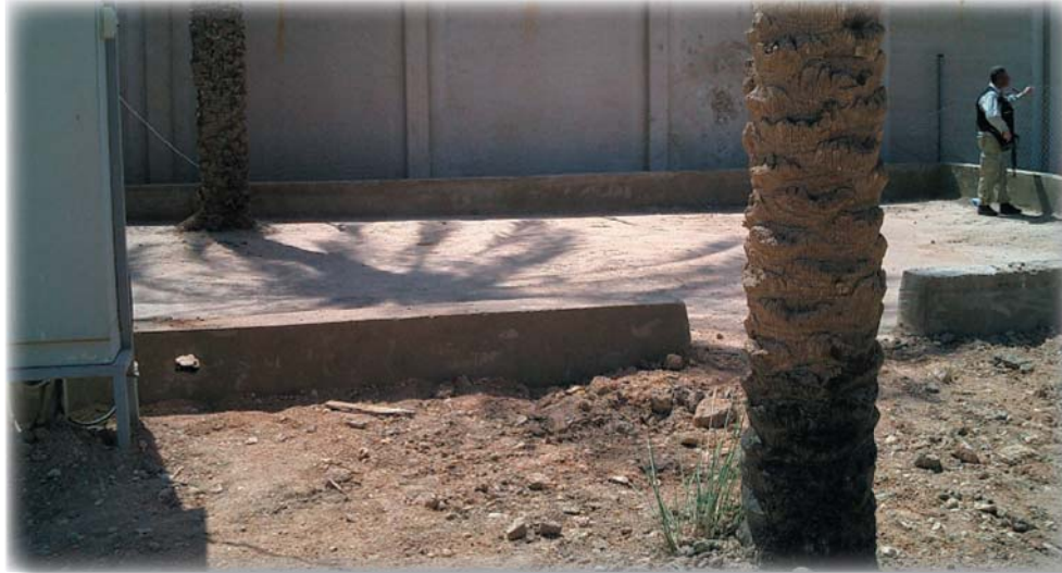
Site for the missing 1-megawatt generator at the Babylon Police Academy.
