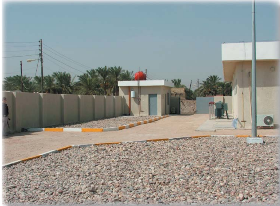
New wall, guardhouse, and gate at electrical facility in central Iraq.
