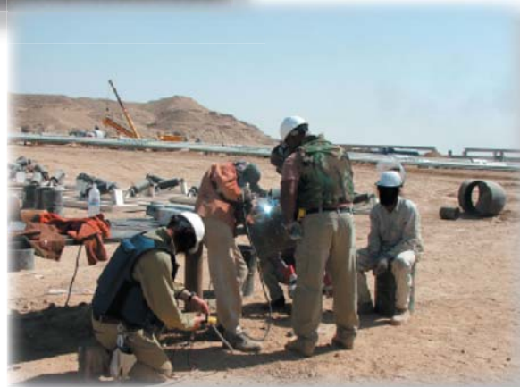
QM team testing a welder's skill at river pipeline crossing site.
