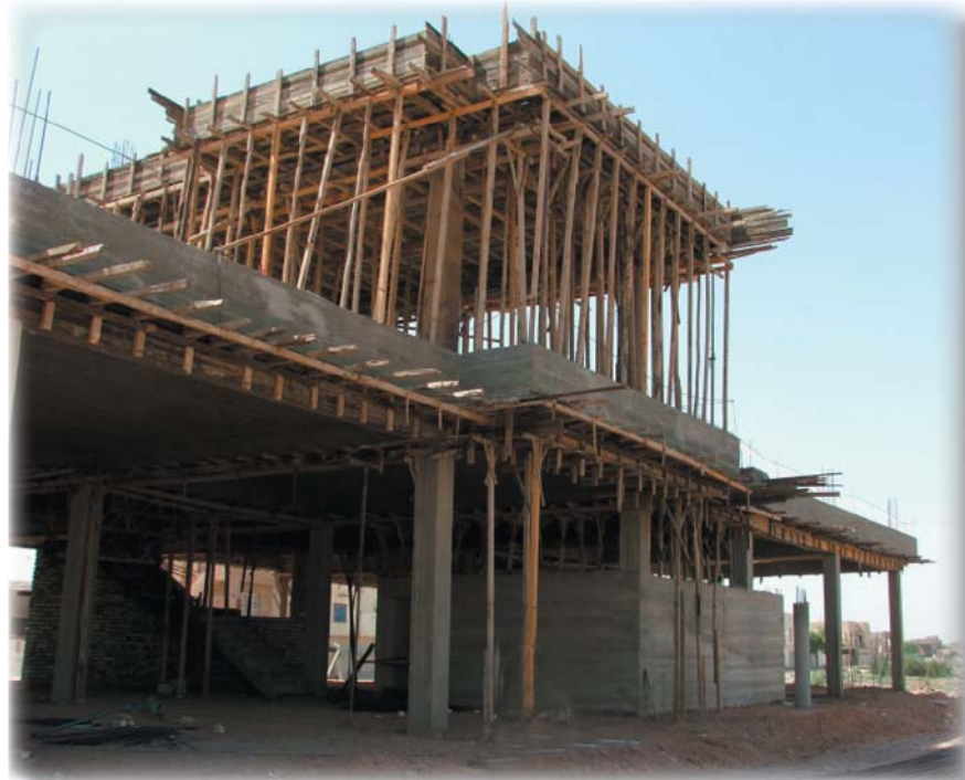
Primary healthcare building in central Iraq, under construction.
