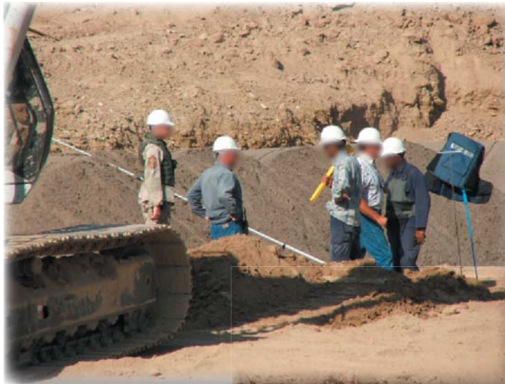
Supervisors on site at river crossing tie-ins.
