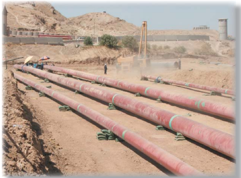
Construction at the tie-in site.
