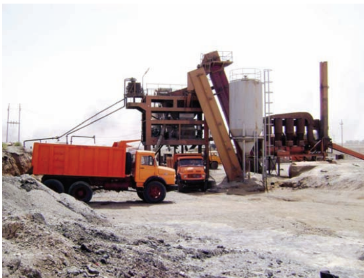
Renovated asphalt plant near Amara. (USACE photo)
