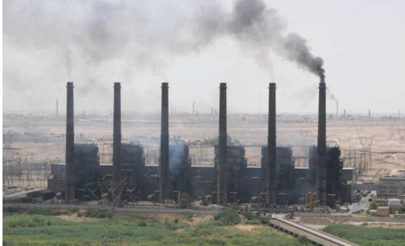
Baiji Power Plant in Salah Al-Din.
