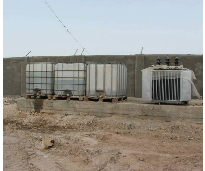
Future generator pad at Al Ager.
