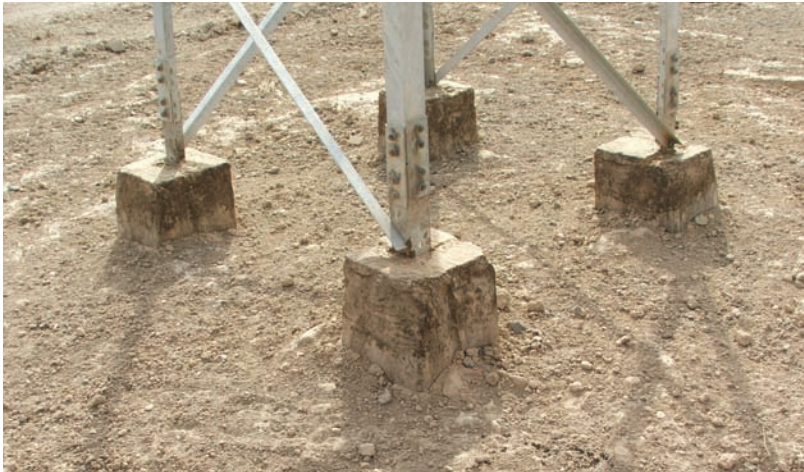
Completed tower foundation on the power line project.
