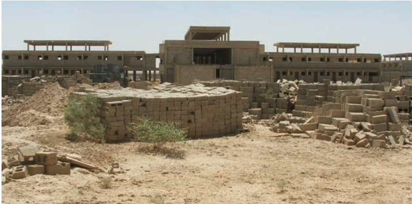
Concrete blocks still onsite at the Kahn Bani Sa'ad Correctional Facility.
