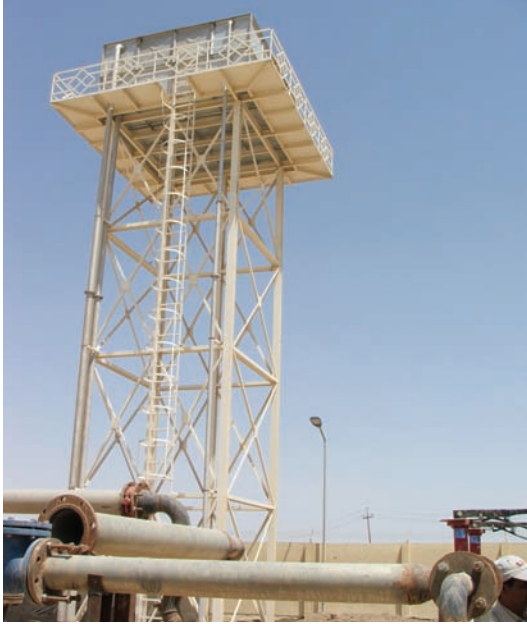
Elevated storage tank at Al Kazim.
