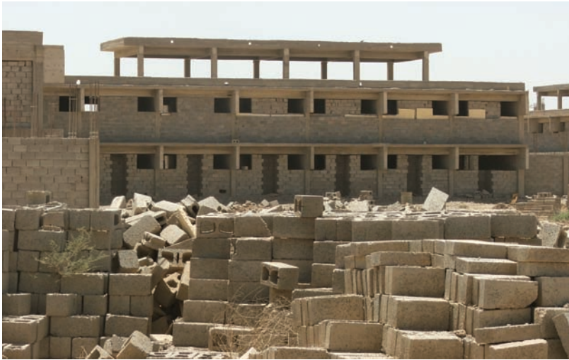
Kahn Bani Sa'ad Correctional Facility: A $40 million project, incomplete and abandoned.
