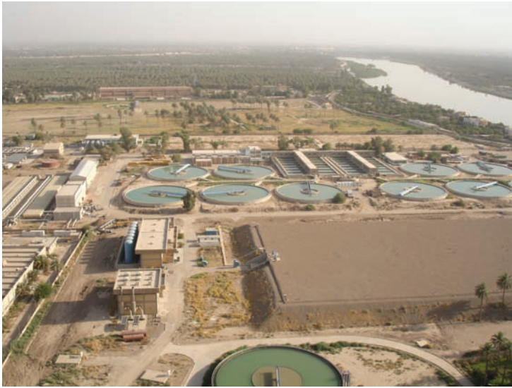
Shark Dijla Water Treatment Plant along Tigris River in northern Baghdad.
