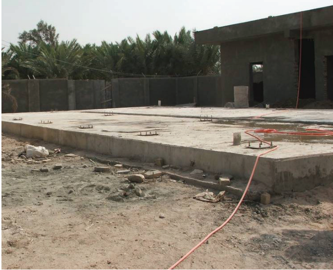
Foundation of the water compact unit at Al Ager.
