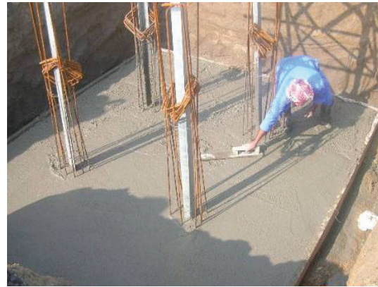
Finishing concrete on the power line project. (USACE photo)
