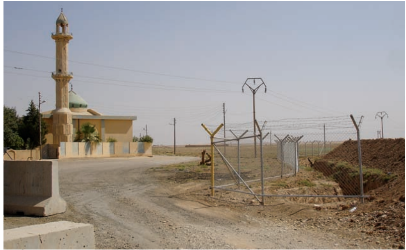
Pipeline Exclusion Zone in Kirkuk: A success story in the resurgence of Iraq's oil industry.
