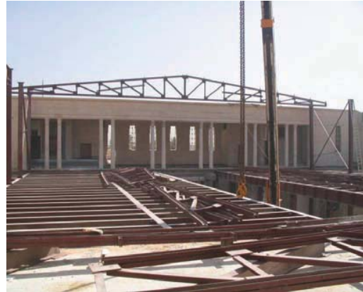
Construction of the third floor (contractor provided photo).
