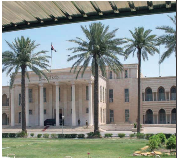
The renovated Iraqi Ministry of Defense headquarters in Baghdad.
