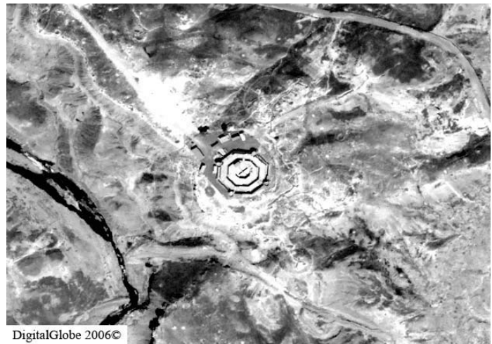
Aerial Image 3. A July 21, 2006 example of the castle style of border forts, which do not fit the "Class C style" border fort, as defined in the contractor-provided blueprints/diagrams.
