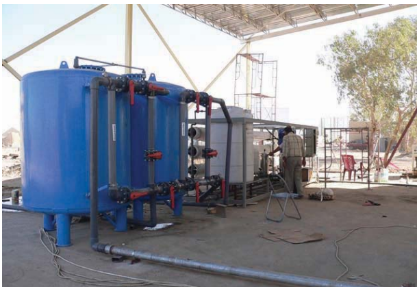
Reverse osmosis unit at installation (contractor-provided photo).
