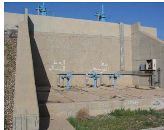
Al Qana'at Raw Water Pump Station.
