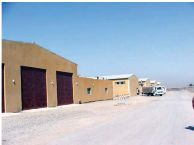
Exterior view of completed 6-bay maintenance shop and 4 warehouse buildings.
