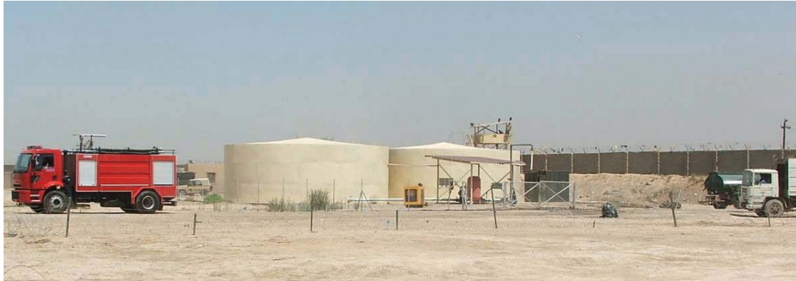
Water tanks at the Al Rasheed Brigade base.
