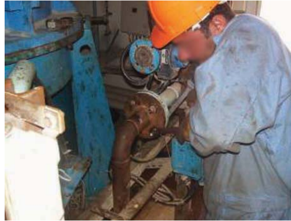
Rehabilitating pumps (picture courtesy of USACE).
