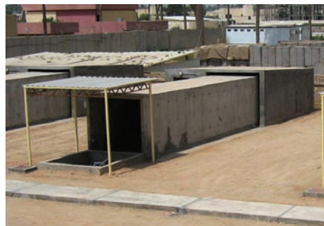
Site Photo 16. Pistol-firing station showing shooter's pit, firing tube, and target enclosure.
