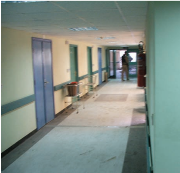
Site Photo 1. Main corridor in women's health and laboratory building.
