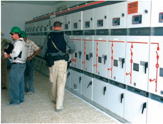
Site Photo 26. Al Hamdan substation distribution: 11 kV switchgear panels at the time of the initial assessment.
