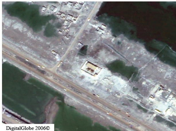
Aerial Image 3. Overview of the Al Hamden electrical substation, which SIGIR personnel visited this quarter.
