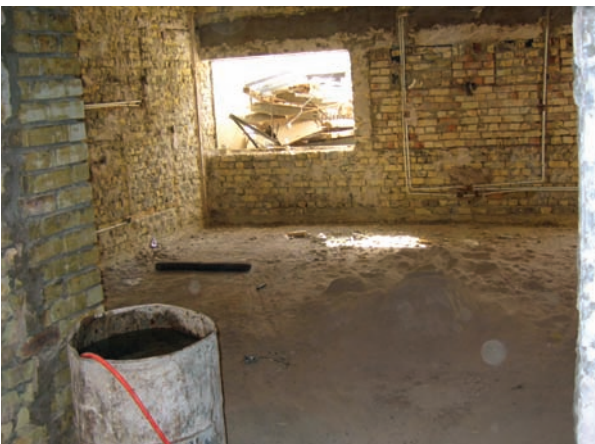
Site Photo 3. Patient ward in Building B9 after demolition of wall plaster and flooring.
