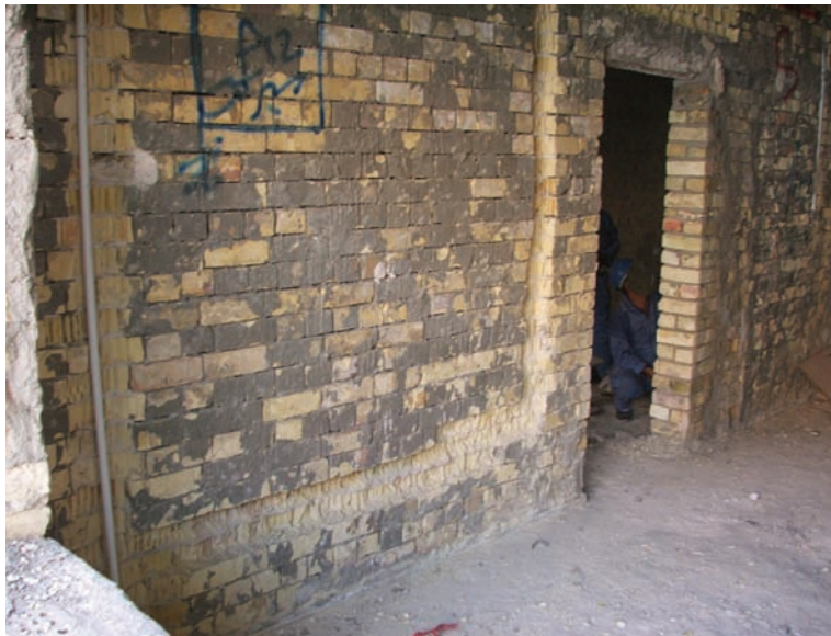
Site Photo 6. Exposed walls in Building B1 before re-plastering.
