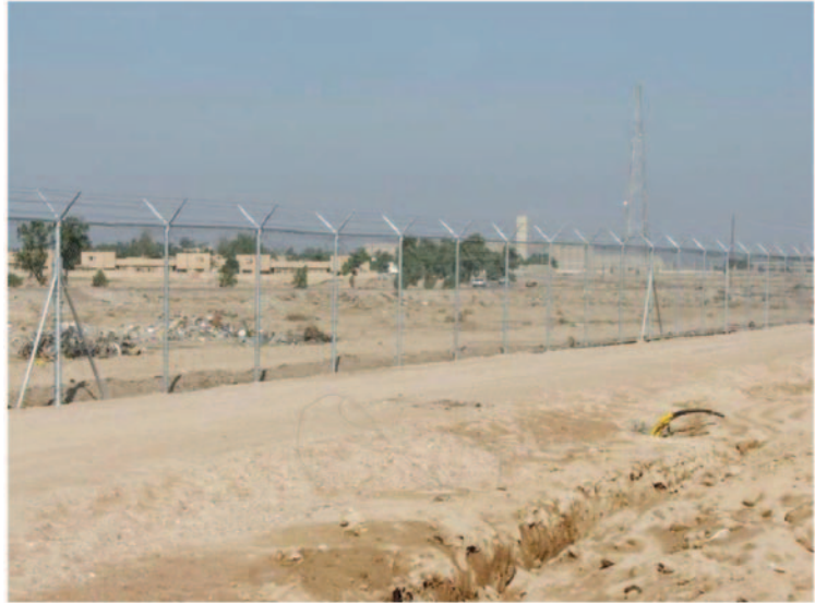
Security fencing and utility trench at Um Qasr
