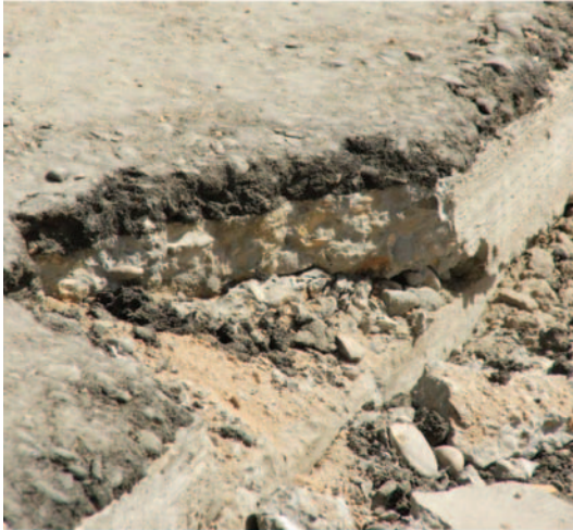
Newly installed concrete and asphalt helicopter pad
