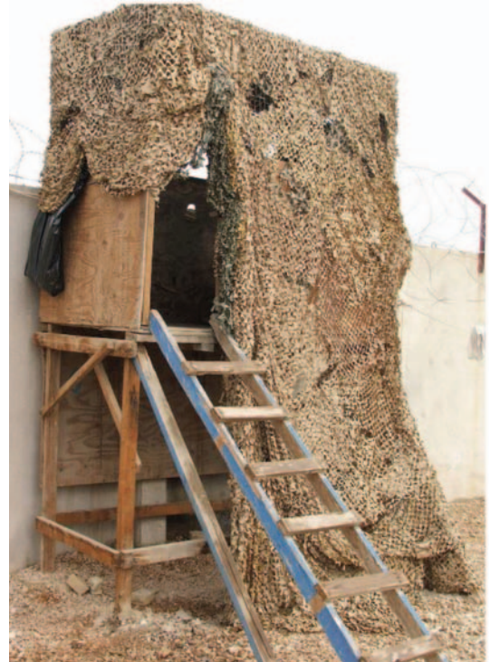
Makeshift Guard Tower at the Hilla Police Academy
