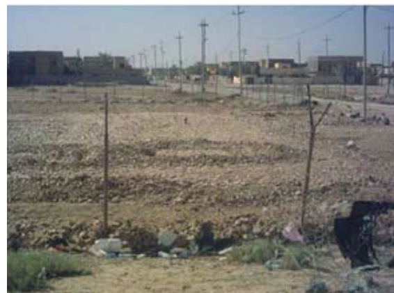
Site 2: after remediation by Parsons
