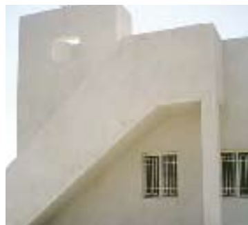
Exterior of checkpoint building
