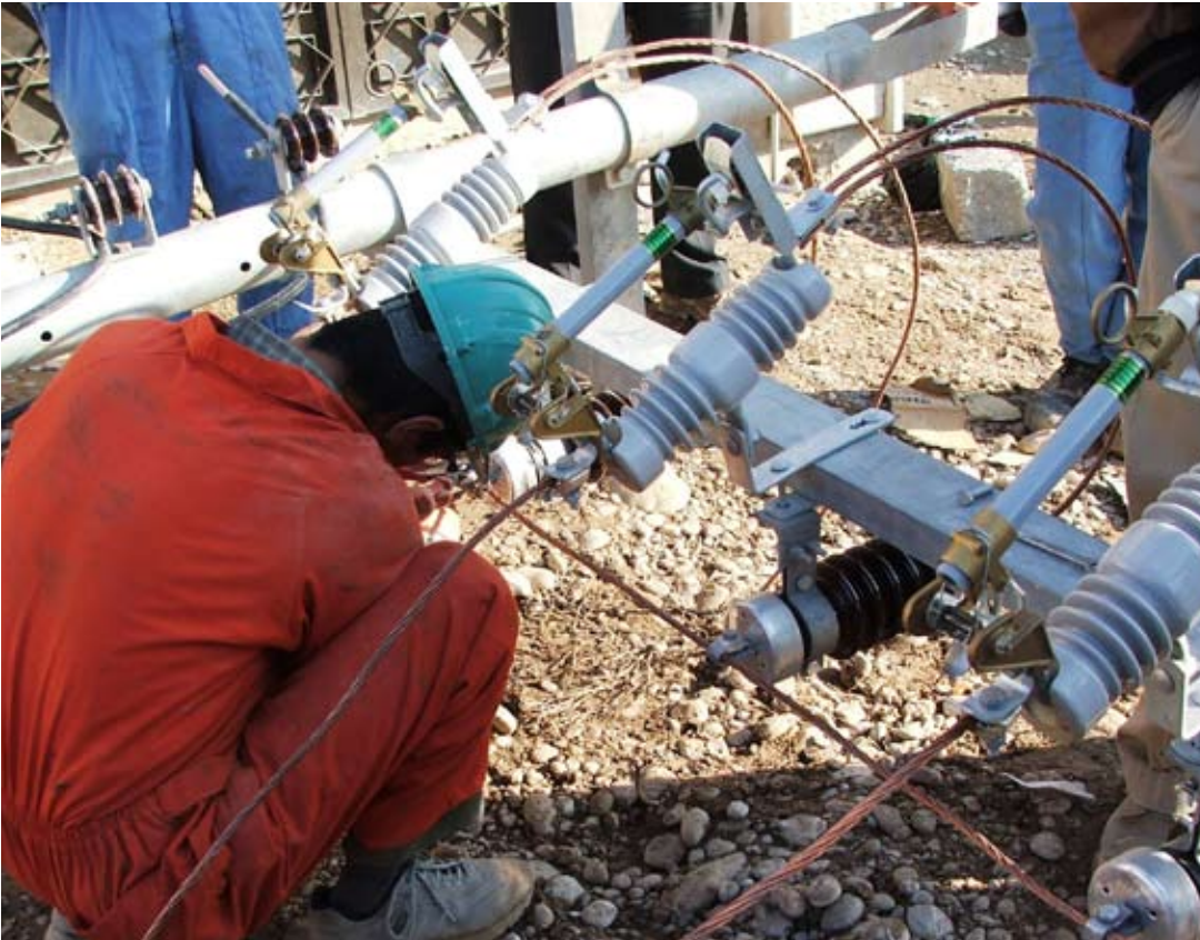
Preparing fuse cutouts on H-pole prior to setting
