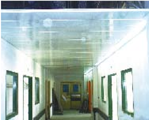
Renovated hallway at one hospital project
