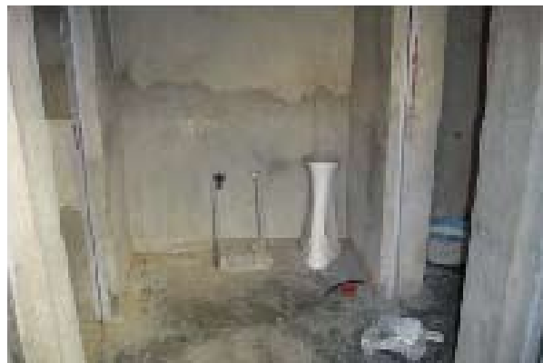
Bathroom fixtures at border post
