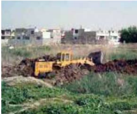
Site 1: before remediation by Parsons
