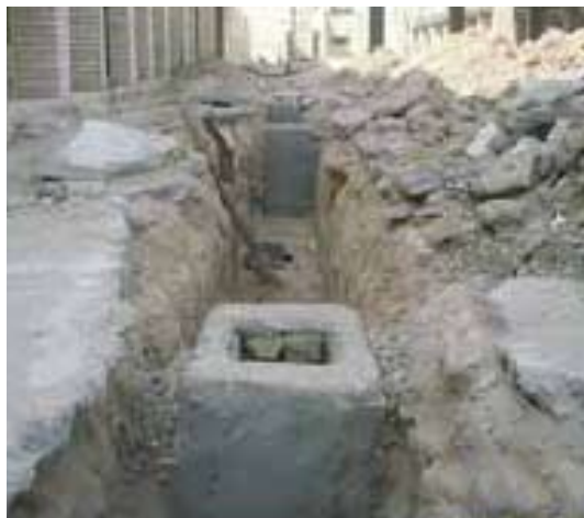
Manholes and excavation work
