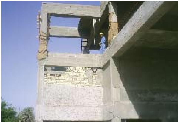
Fire station under construction
