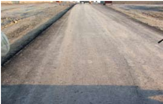
Asphalt concrete pavement near village of Balawat
