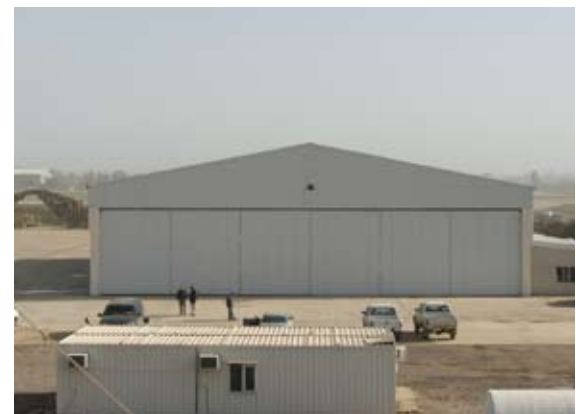
Exterior view of aviation hangar
