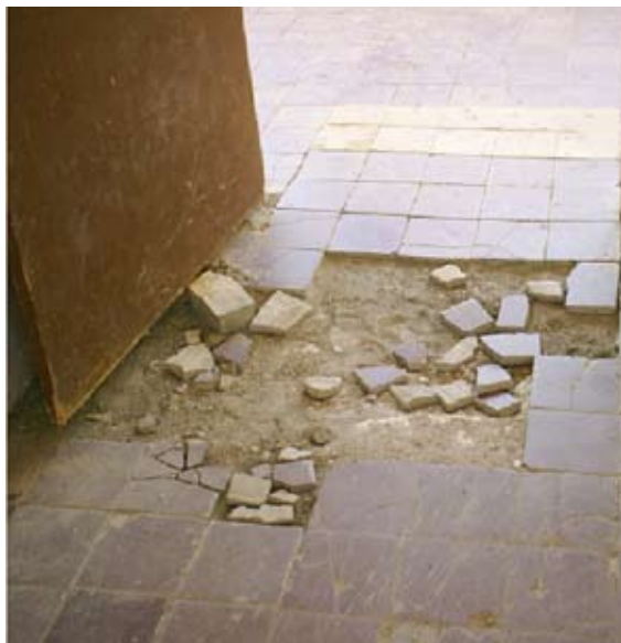
Broken tiles in school classroom
