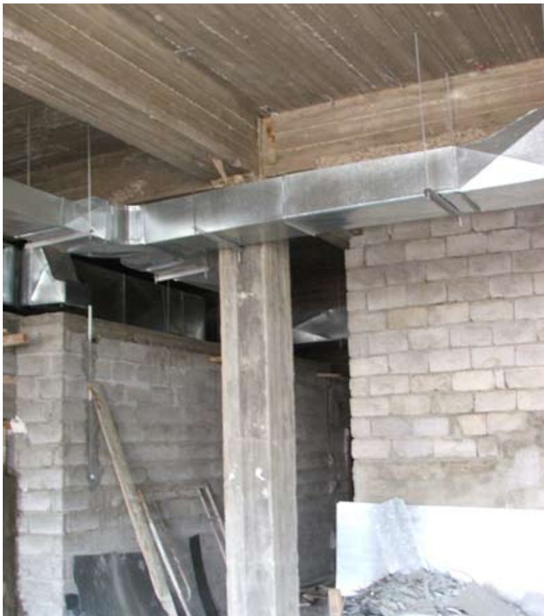
Reinforced load-bearing column out of plumb
