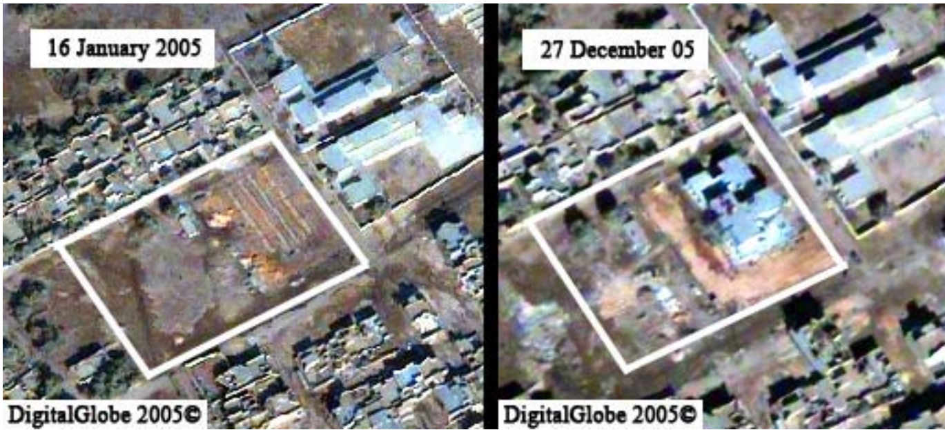
Images 5 and 6. Comparison of imagery showing progress made at a public health clinic in southern Iraq between January 16, 2005 (left) and December 27, 2005 (right). The image on the left shows the initial ground preparation for construction. The image on the right shows the final leveling of soil around the clinic, which was noted as a deficiency in an earlier Ground Project Survey visit.
