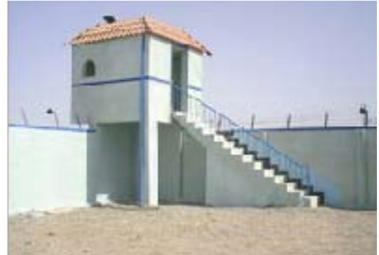
Perimeter security wall with concertina wire and guard post
