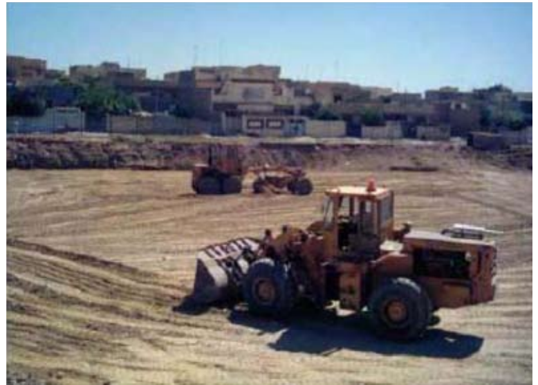
Site 1: after remediation by Parsons
