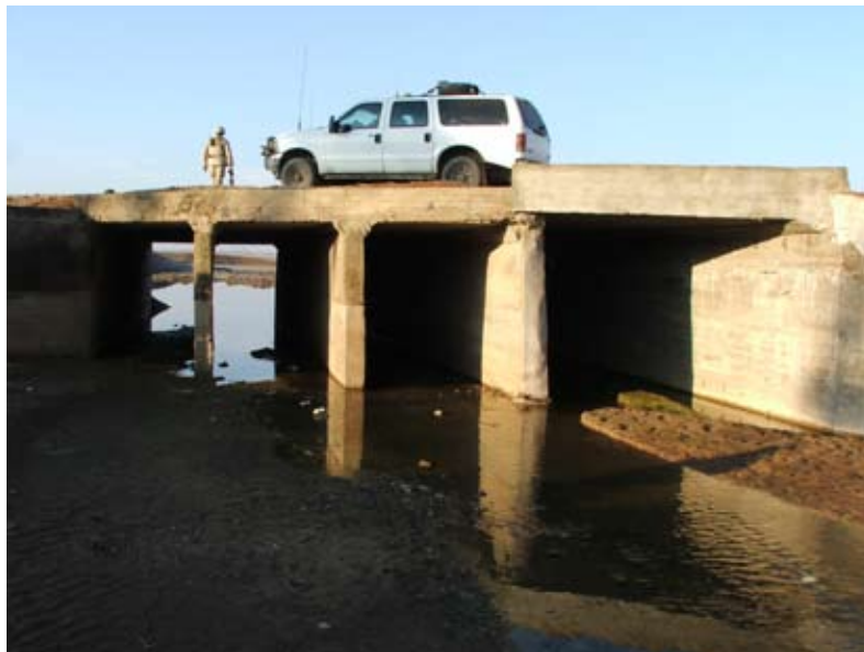
Extension of existing box culvert
