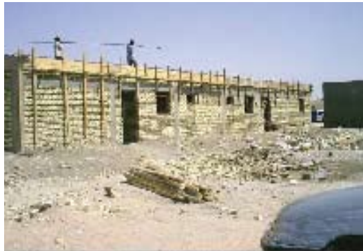
Police Station construction
