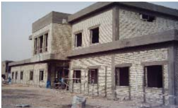
Exterior front of a primary health care clinic
