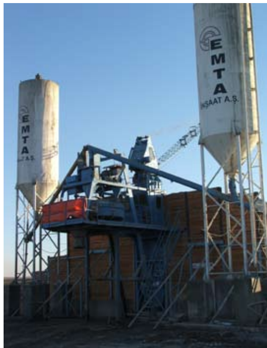
Concrete batch plant to mix concrete
