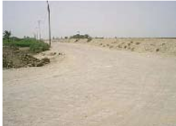
Graded surface of Thi-Qar road project
