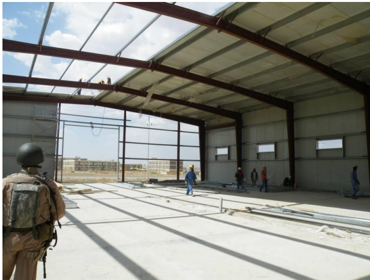
Site Photo 6. Maintenance garage prior to completion of exterior panel installation
