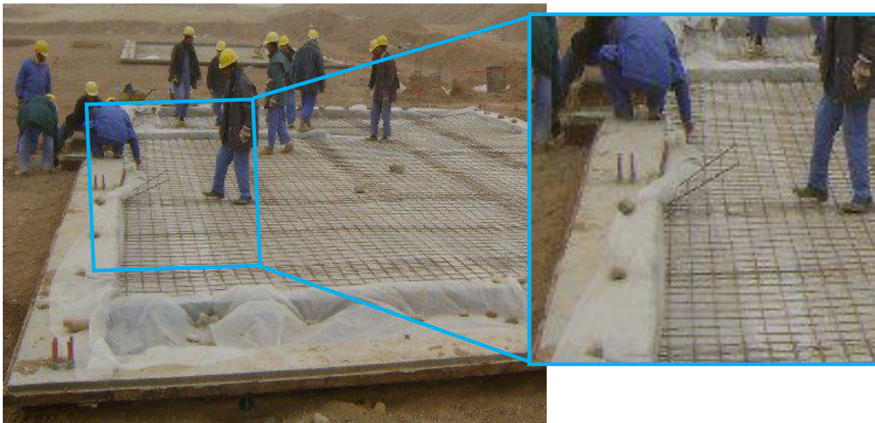
Site Photo 13. Hairpin placement (Courtesy of USACE)
