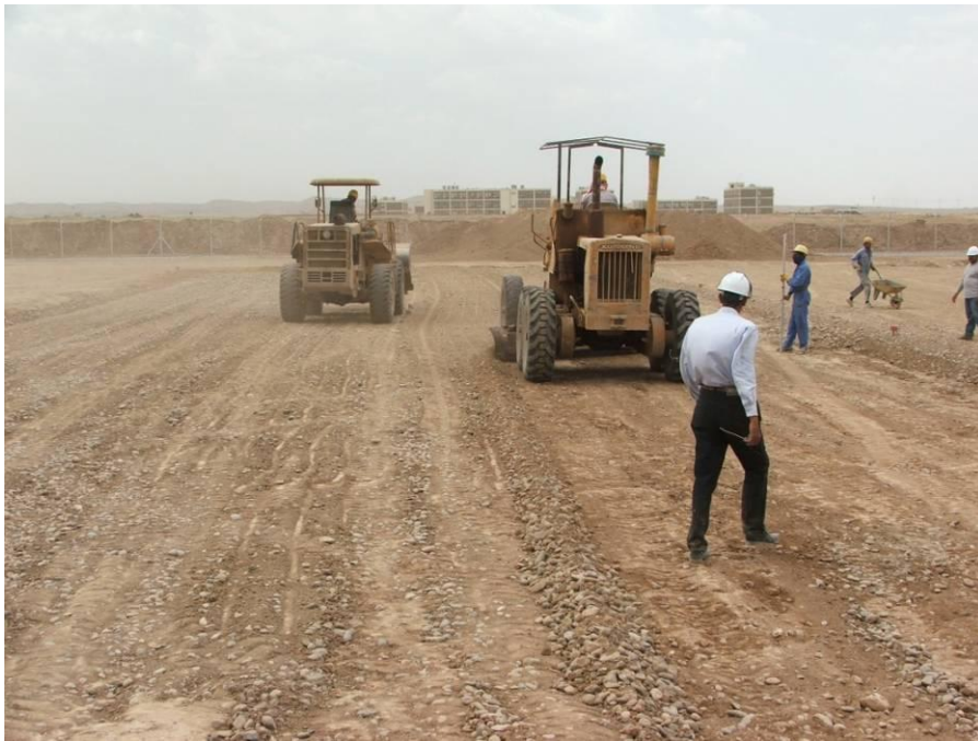
Site Photo 11. Site grading for diesel storage at the distribution point
