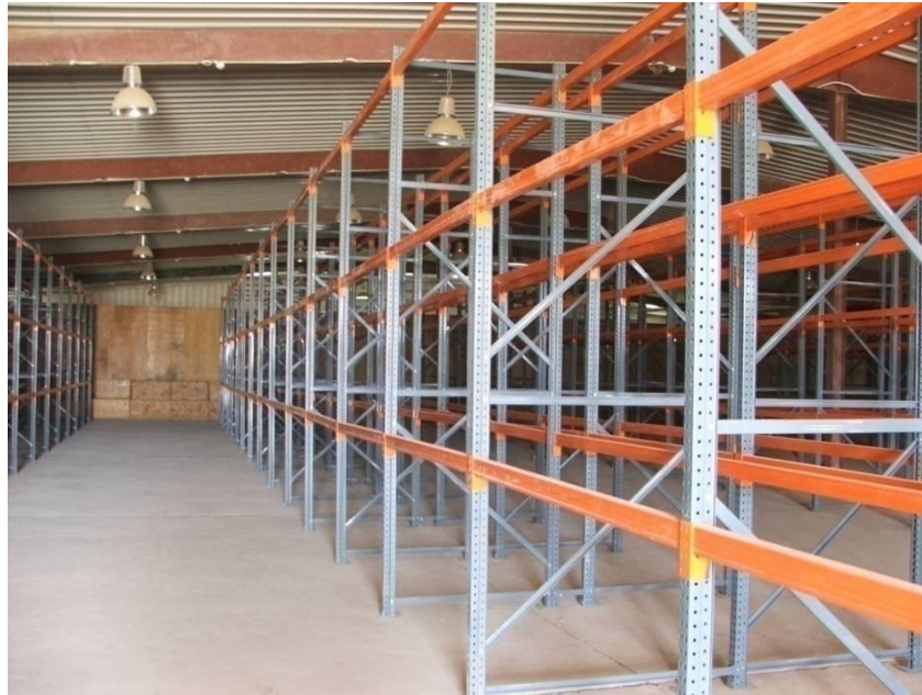
Site Photo 5. Pallet racks in existing warehouse
