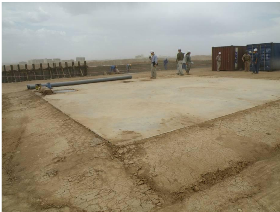
Site Photo 10. Completed tank foundation
