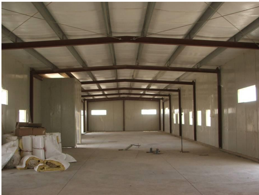
Site Photo 2. Warehousing platoon administration building interior
