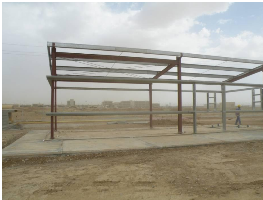
Site Photo 9. Office building
