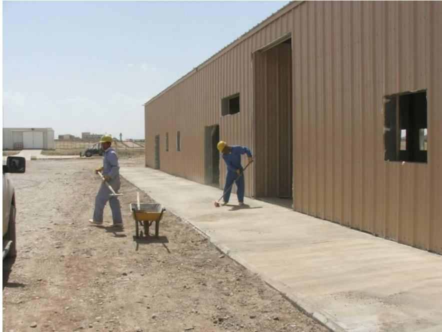
Site Photo 1. Site grading at the front of the administration building
