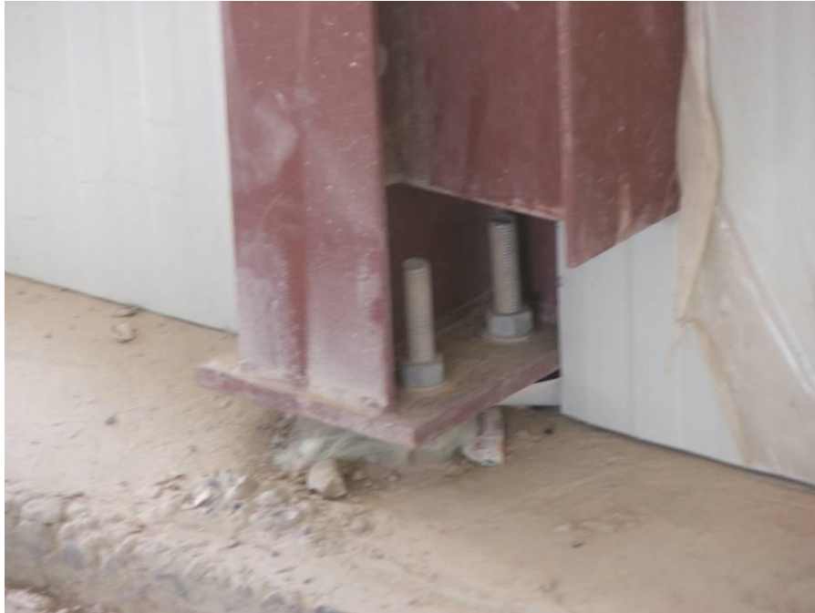
Site Photo 3. Column base plate prior to placement of non-shrink grout
