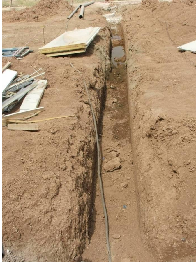
Site Photo 7. Electric utility trench
