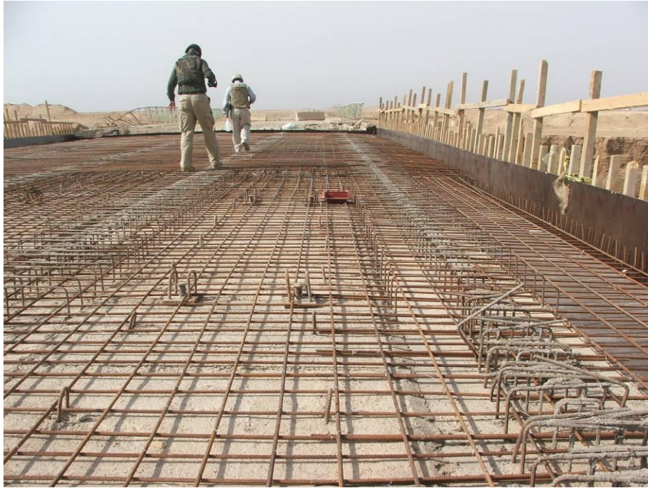
Site Photo 7. Concrete deck reinforcing (prior to placing top mat, foreground)
