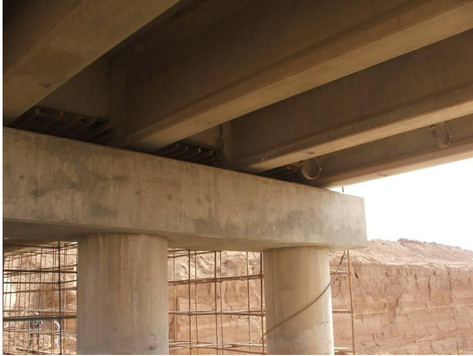
Site Photo 15. Bent cap at Pier No. 1
