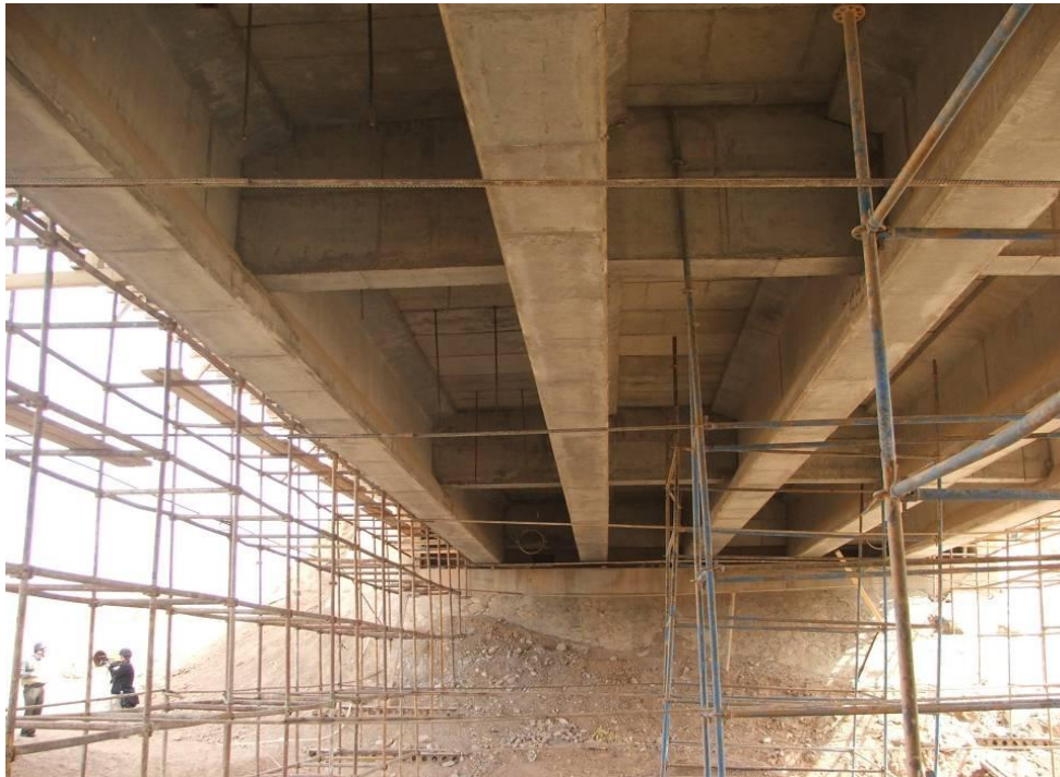
Site Photo 10. Post-tensioned concrete girders
