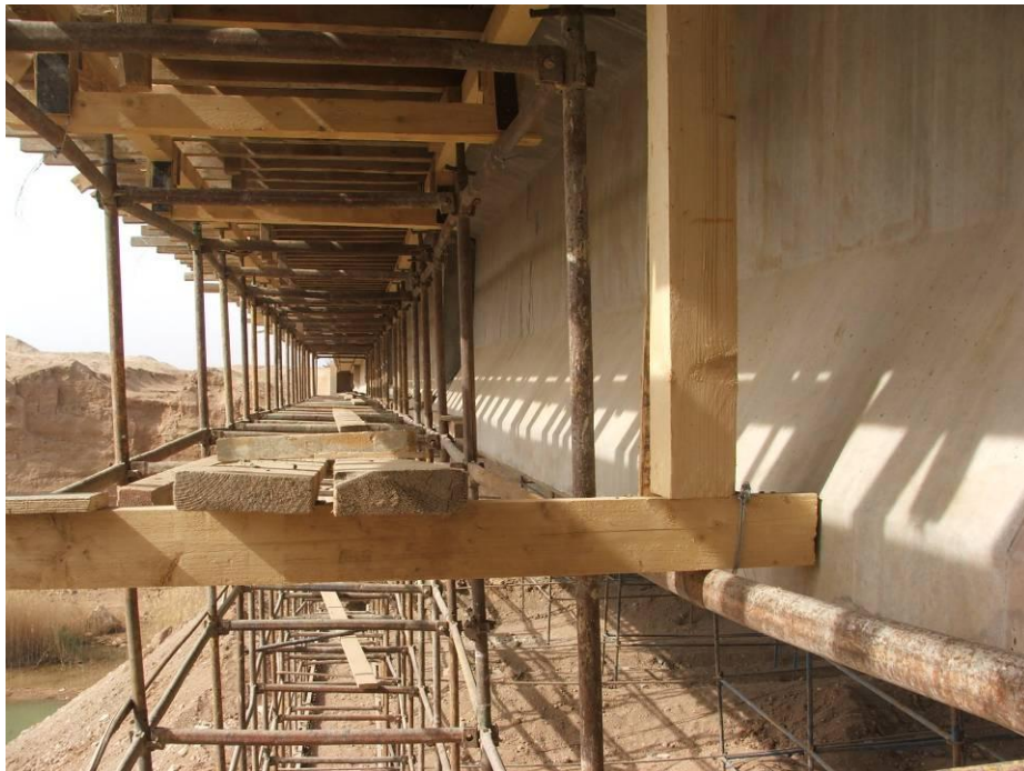
Site Photo 8. Falsework for forming concrete deck overhang
