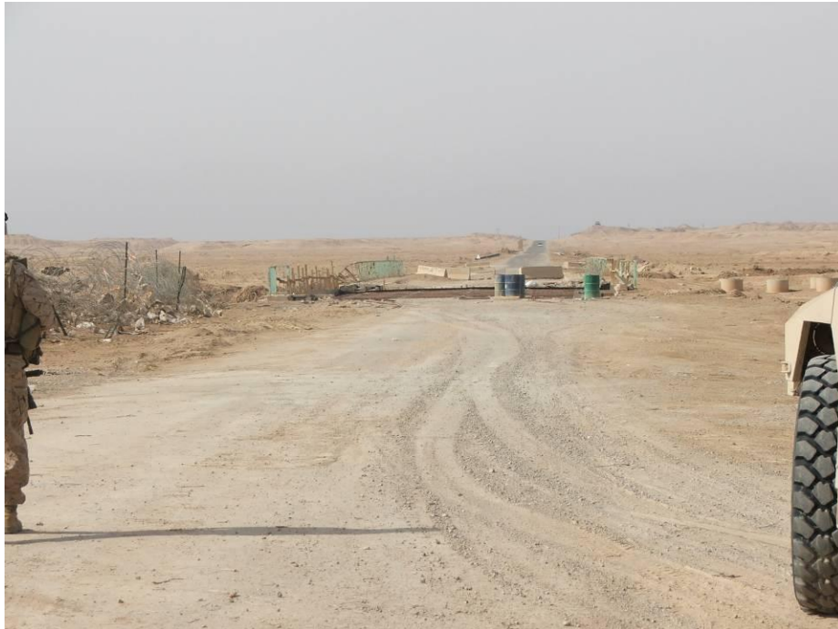
Site Photo 5. Northern approach roadway looking south across the bridge
