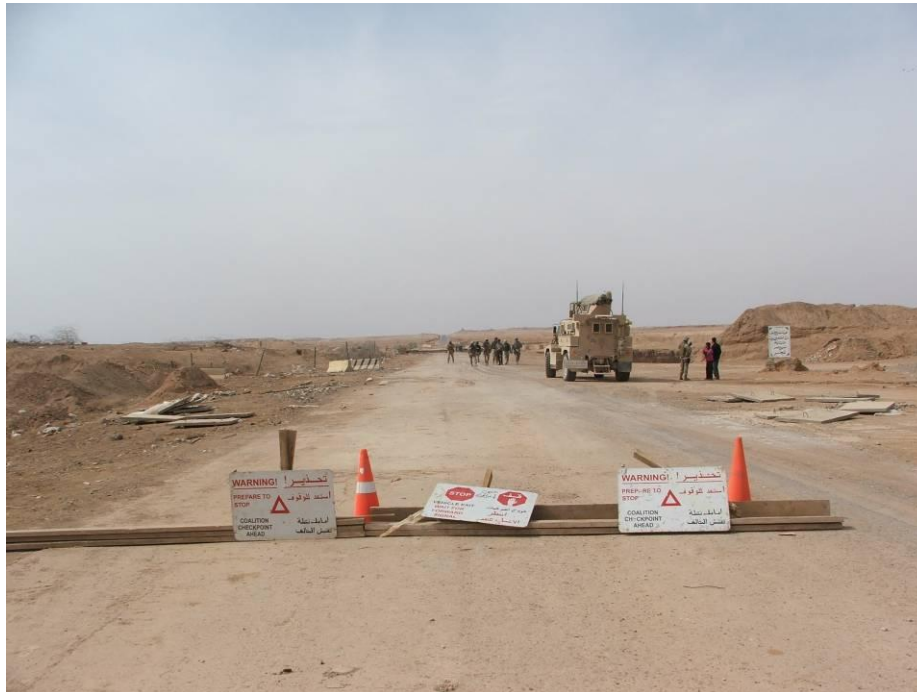
Site Photo 6. Traffic control signs looking south across the bridge
