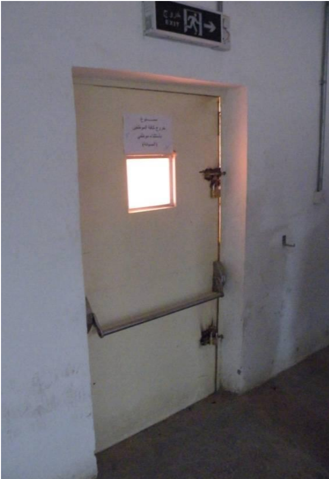
Site Photo 16. Newly installed security door funded by the IHT
