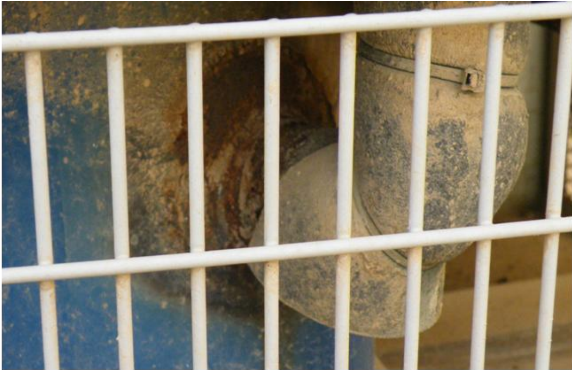
Site Photo 13. Welding done on HVAC unit
