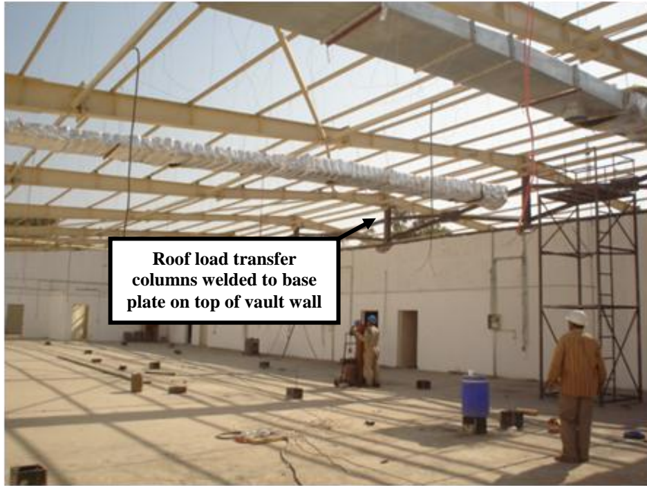
Site Photo 3. Base plate and columns (Courtesy of GRC)
