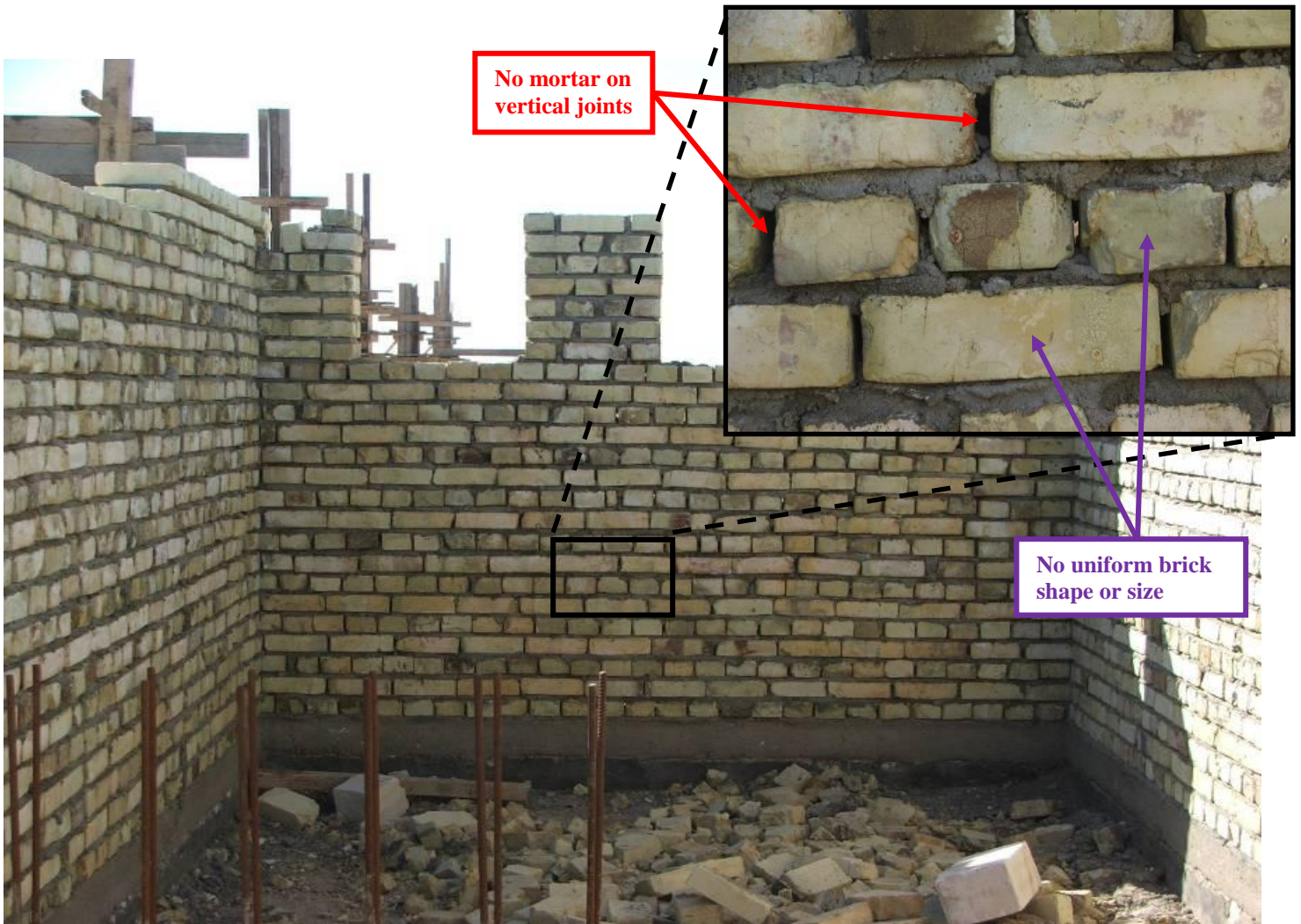
Site Photo 18. Physicians' residence (typical example of brick construction)
