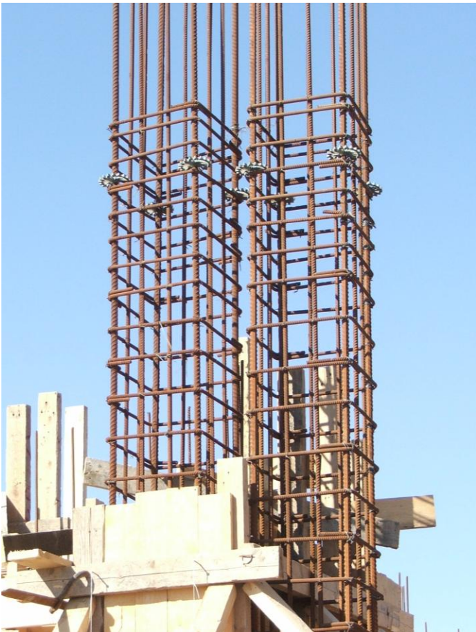
Site Photo 14. Double column forming
