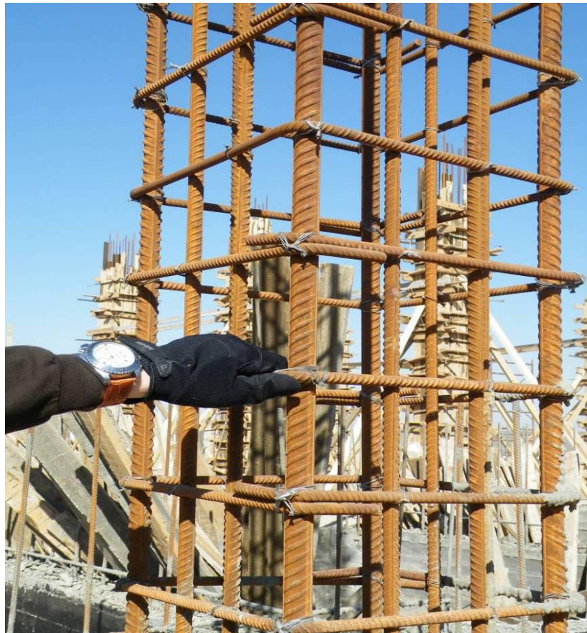
Site Photo 5. Example of constructed column section
