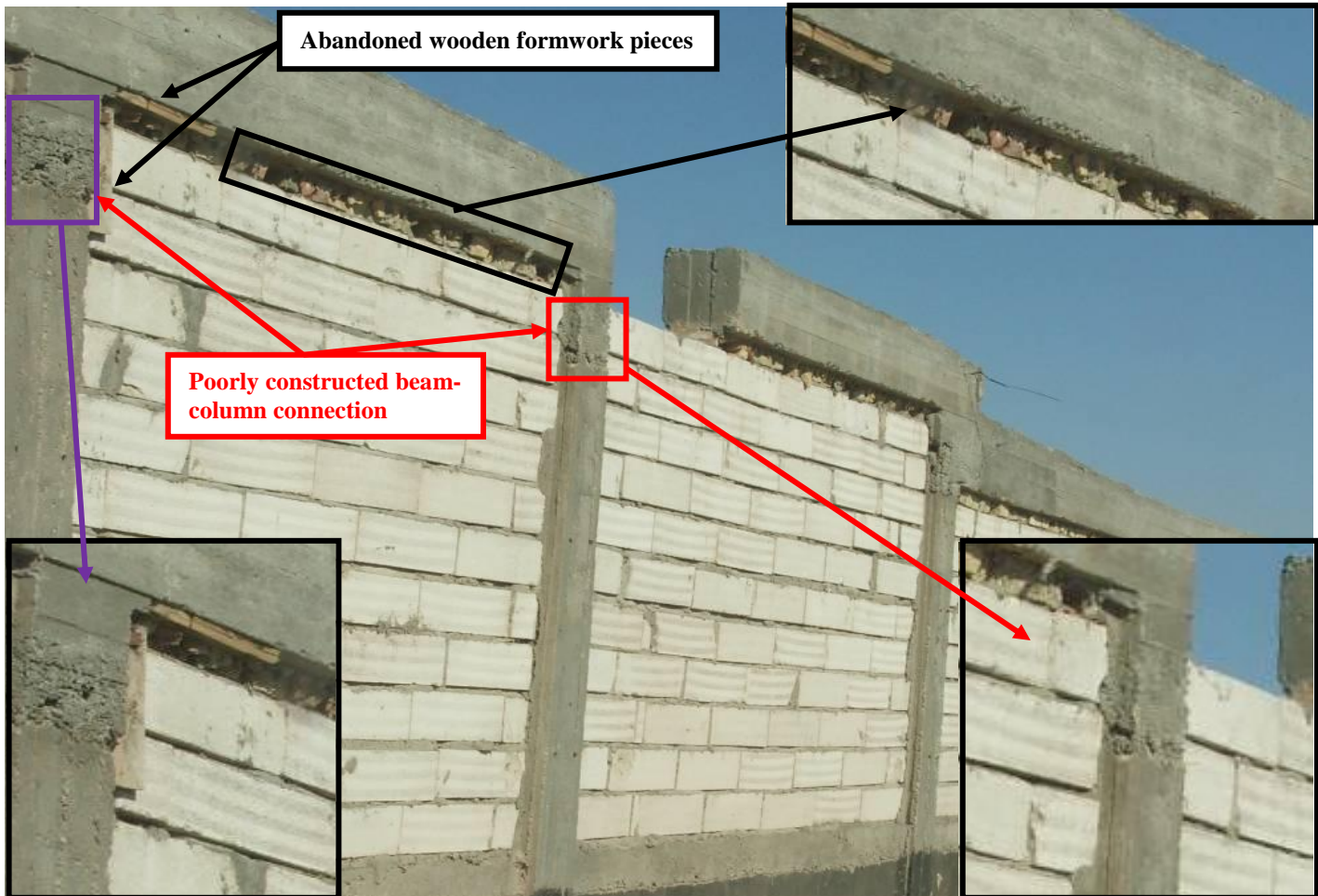
Site Photo 3. Perimeter security wall construction
