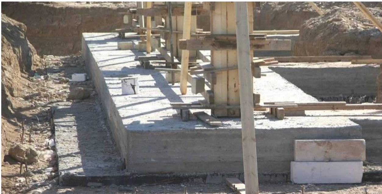
Site Photo 11. Foundation prior to backfill
