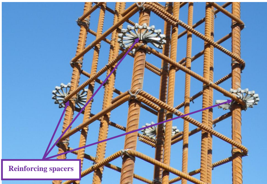
Site Photo 6. Column reinforcing cage and form spacers
