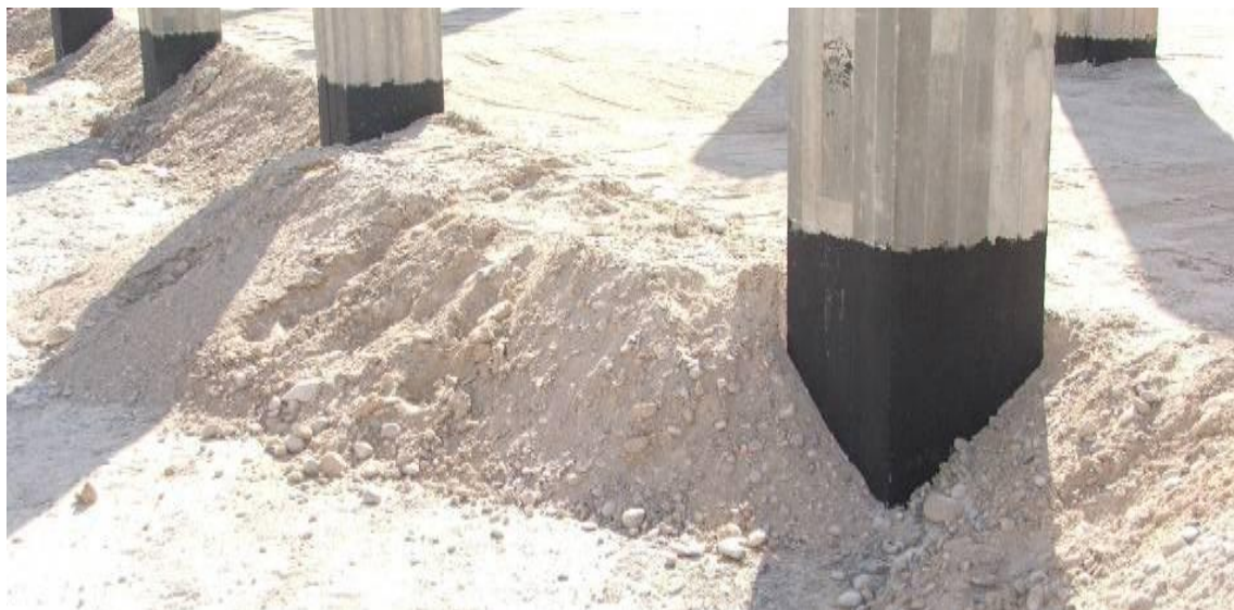
Site Photo 12. Edge of backfill over foundation
