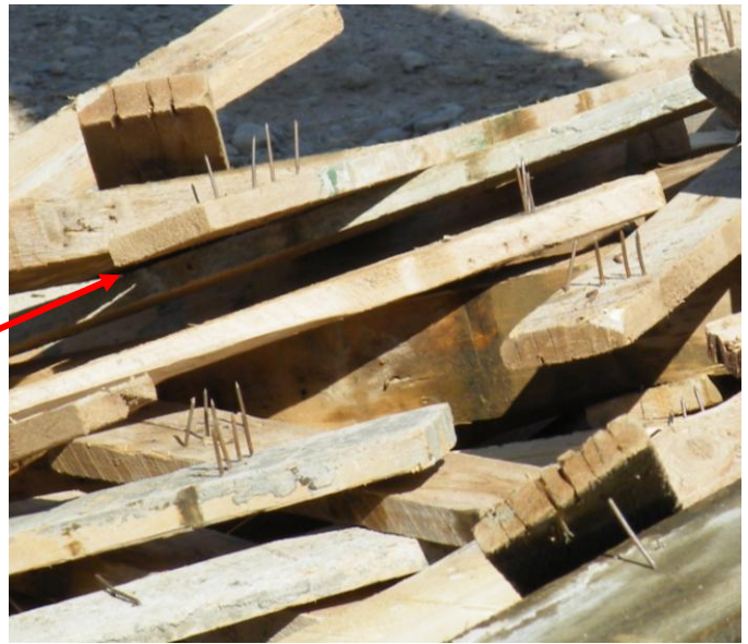
Site Photo 22. Enlarged portion of Site Photo 21
