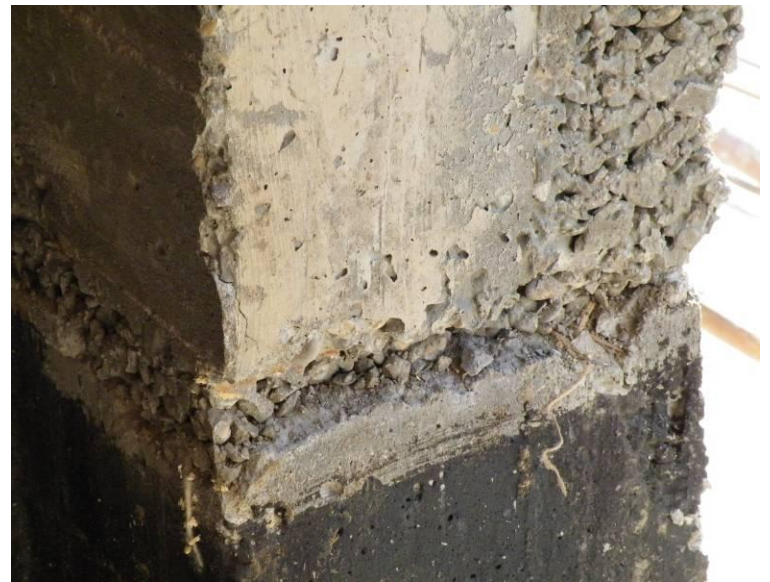
Site Photos 7 and 8. Typical examples of slight to moderate concrete honeycombing in columns
