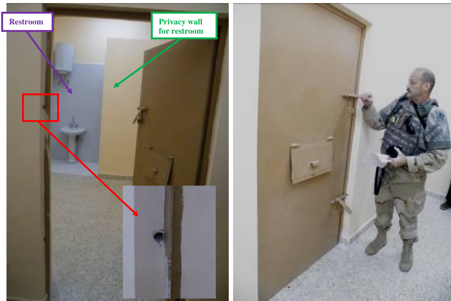
Site Photos 16 and 17. Holding cell door and locking mechanism
