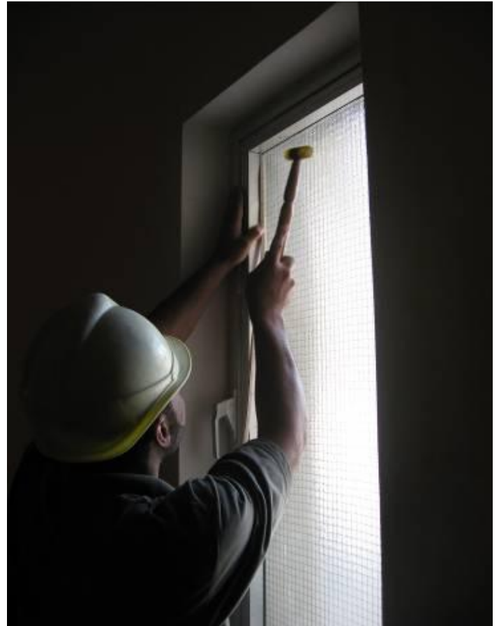
Site Photo 6. Installation of ballistic glass for windows (Courtesy of GRS)
