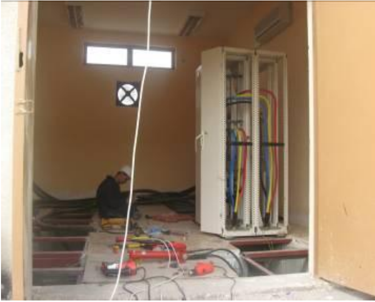
Site Photos 3 and 4. Installation of electrical wiring and mosaic tile, respectively (Courtesy of GRS)
