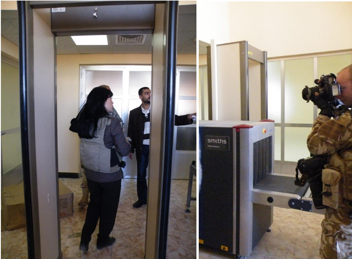
Site Photos 22 and 23. Courthouse building metal detector and scanner
