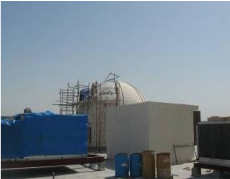
Site Photo 5. Stone covering process for the courthouse dome (Courtesy of GRS)
