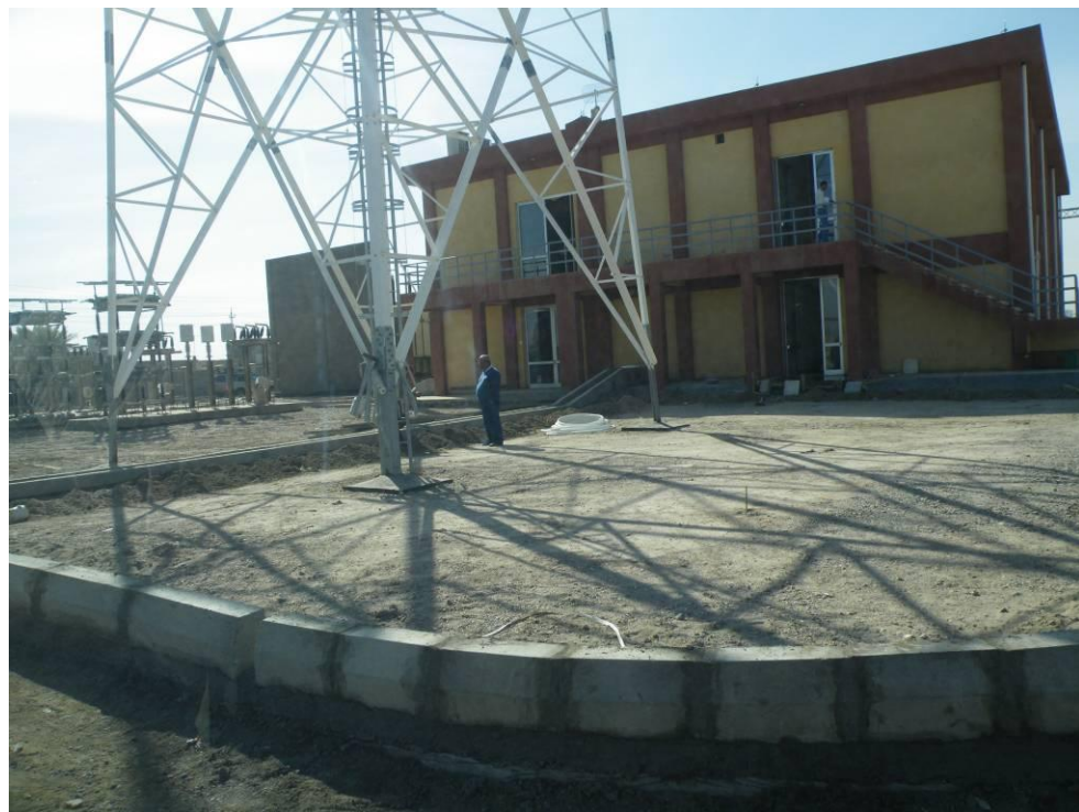
Site Photo 15. Communications tower
