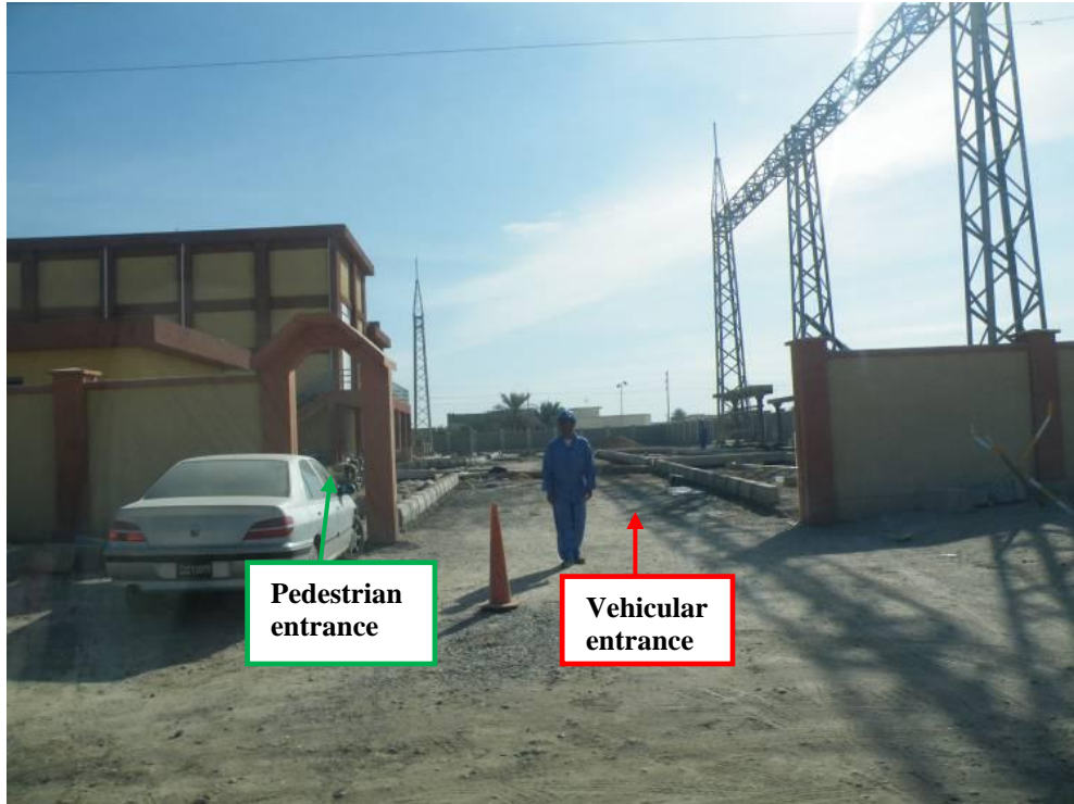
Site Photo 17. Pedestrian and vehicular entrances
