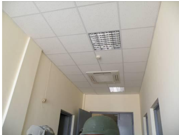
Site Photo 5. Interior finish
