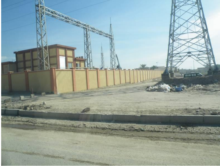
Site Photo 2. Exterior perimeter wall
