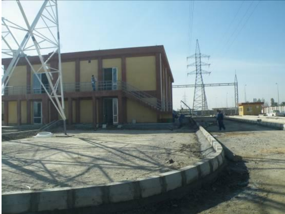
Site Photo 4. Exterior substation building
