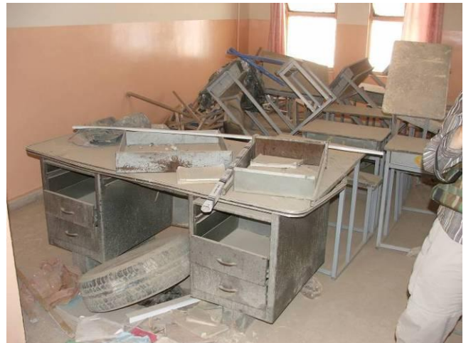
Site Photo 44. Unfinished 2 nd floor (Al Faoo)
