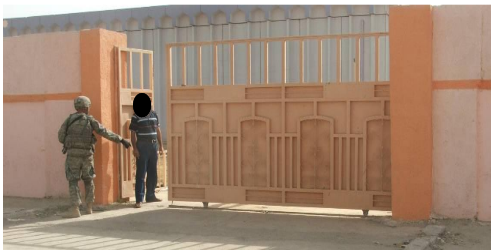
Site Photo 31. Exterior fence and gate (Al Faoo)
