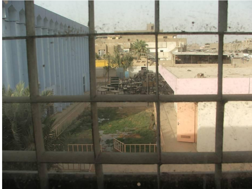
Site Photo 32. No screens in windows (Al Quds)
