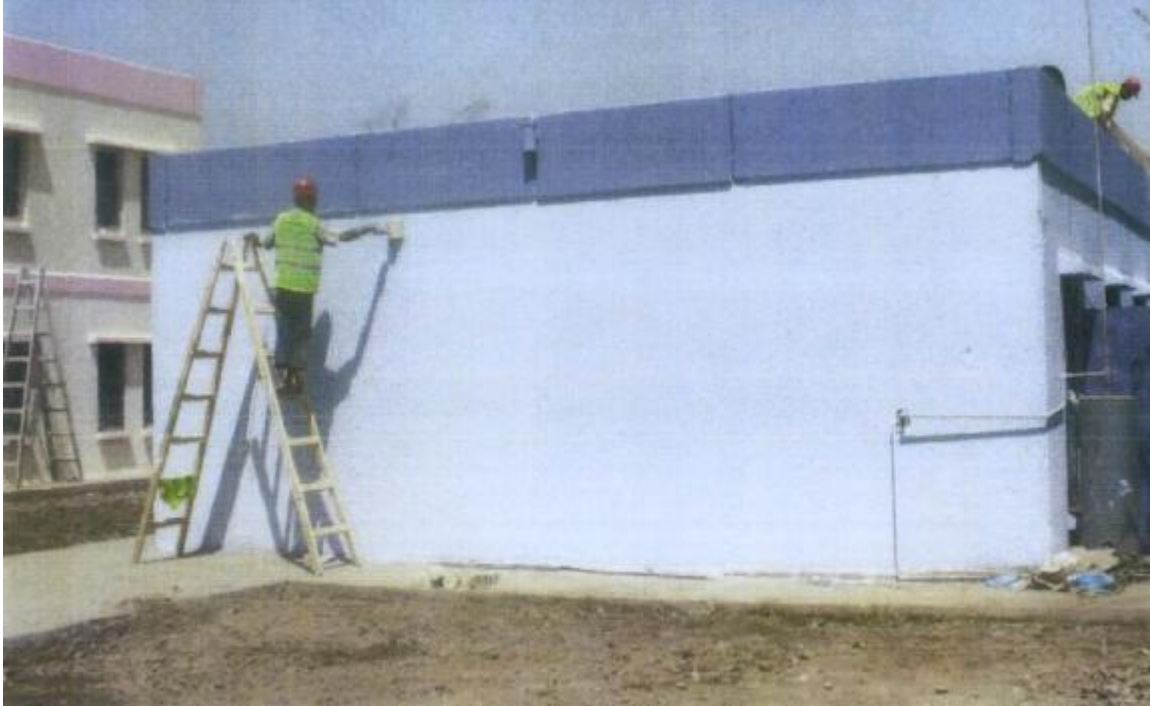
Site Photo 2. Exterior painting at Al Quds (Photo courtesy of MNC-I)
