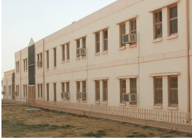
Site Photo 14. Painted exterior (Al Faao)
