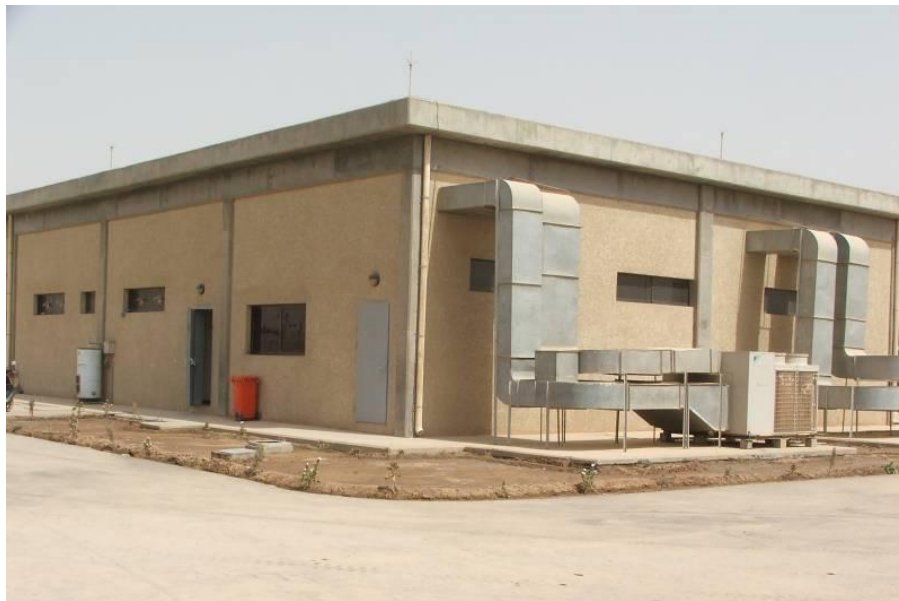
Site Photo 5. Operator building
