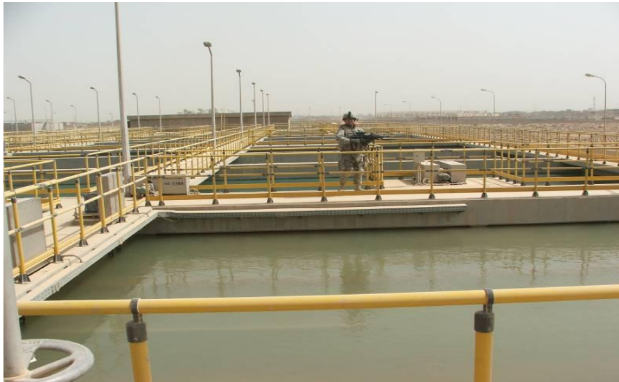
Site Photo 13. Flocculation tanks
