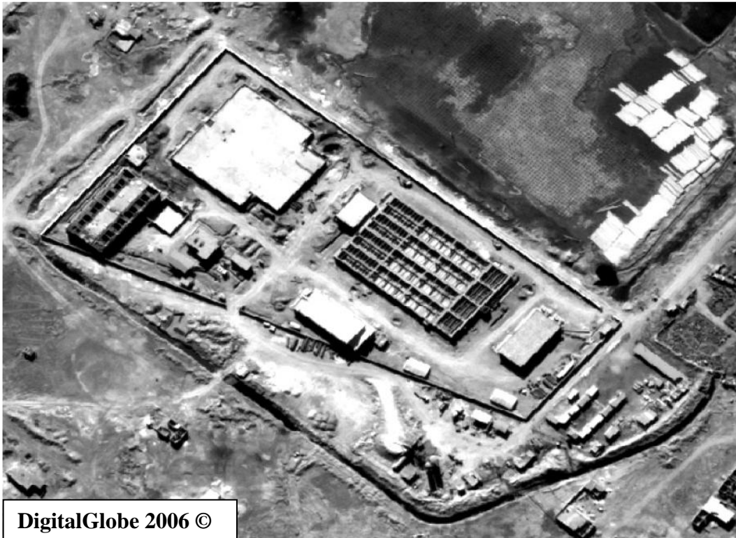
Aerial Image 1. Sadr City Water Treatment Plant in November 2006
