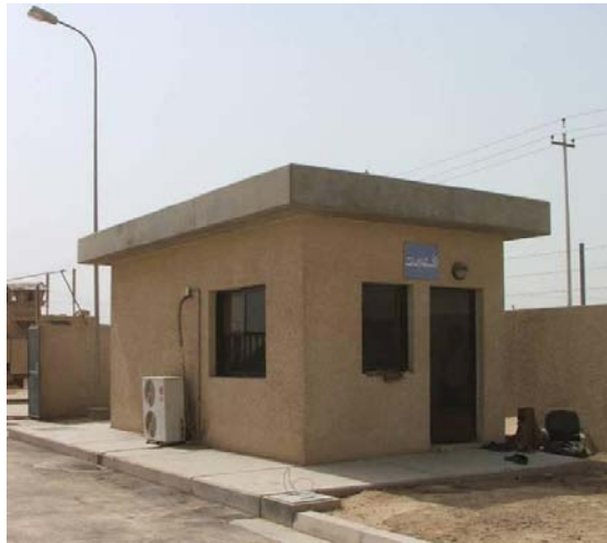
Site Photo 1. Guard building
