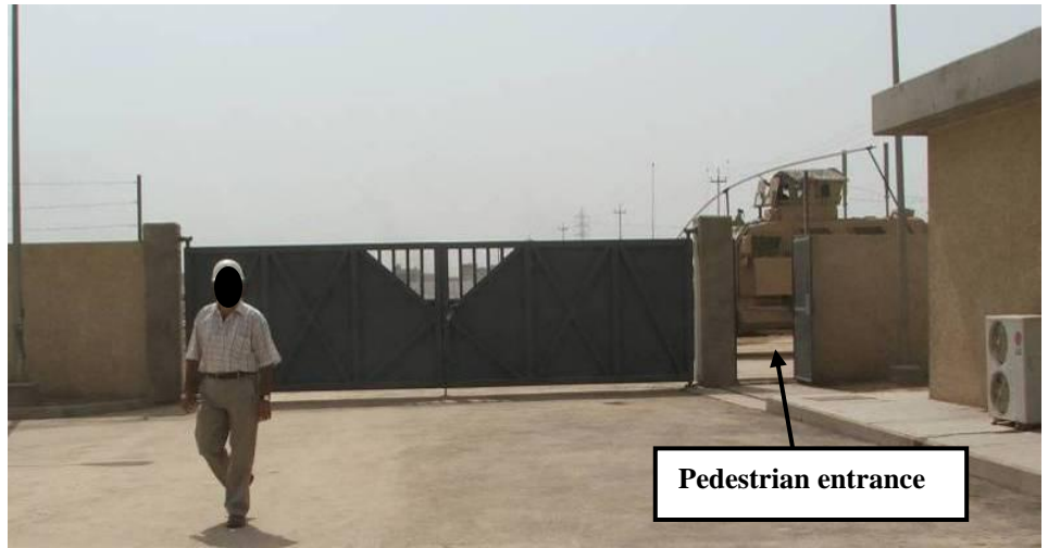
Site Photo 4. Perimeter gate (with pedestrian entrance)
