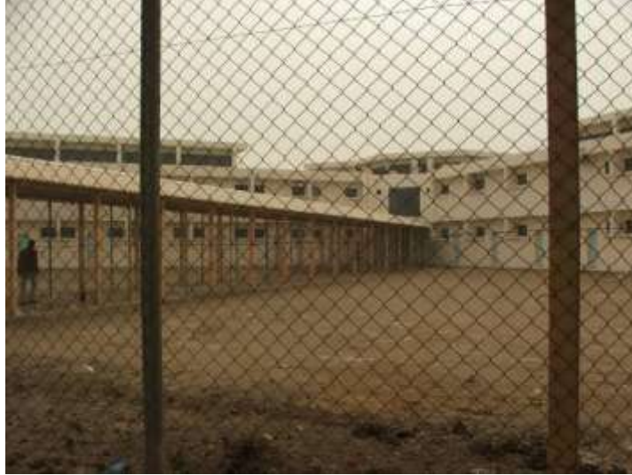
Site Photo 3. Entrance and walkway of inmate housing
