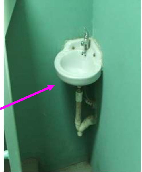
Site Photo 7. Prison cell sink
