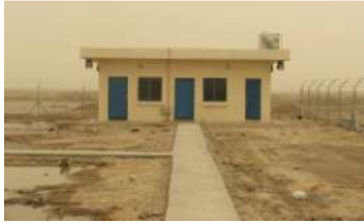
Site Photo 25. STP Administrative building
