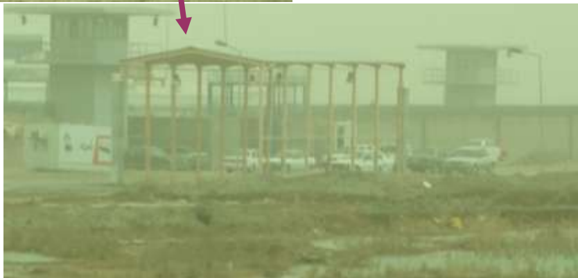
Site Photos 22 and 23. Covered search pit and close-up
