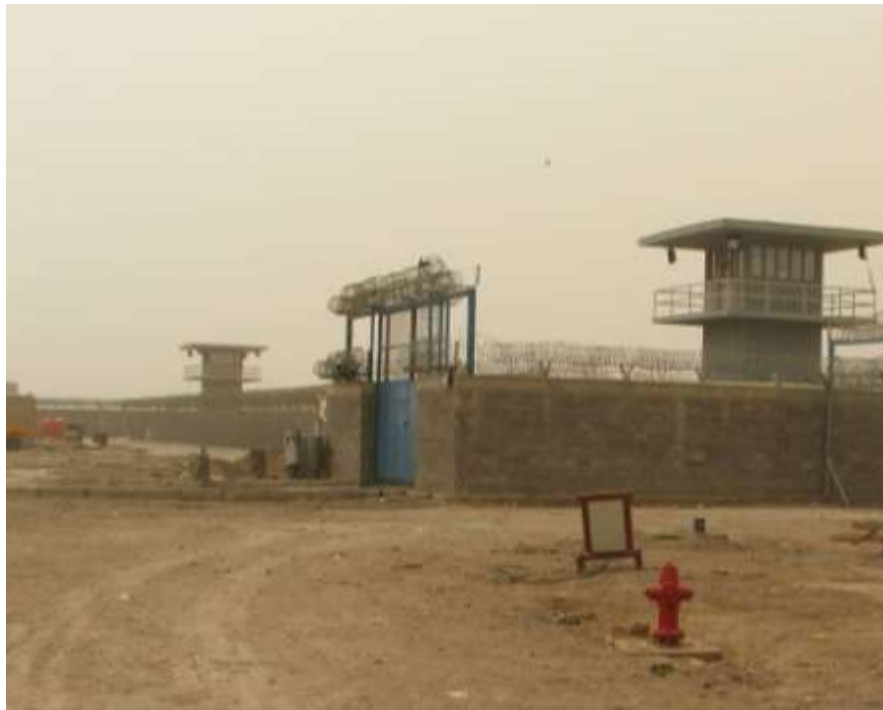
Site Photo 2. Sully gate, guard tower, perimeter wall and interior chain link fences along prison perimeter.
