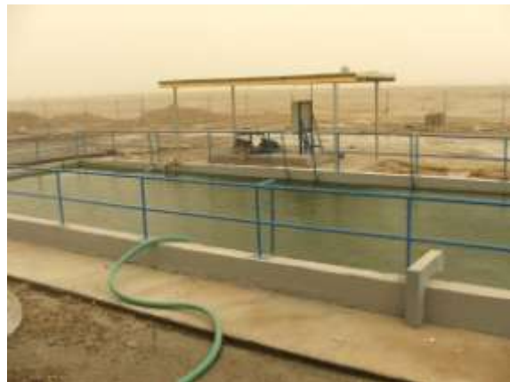
Site Photo 26. Settling tank
