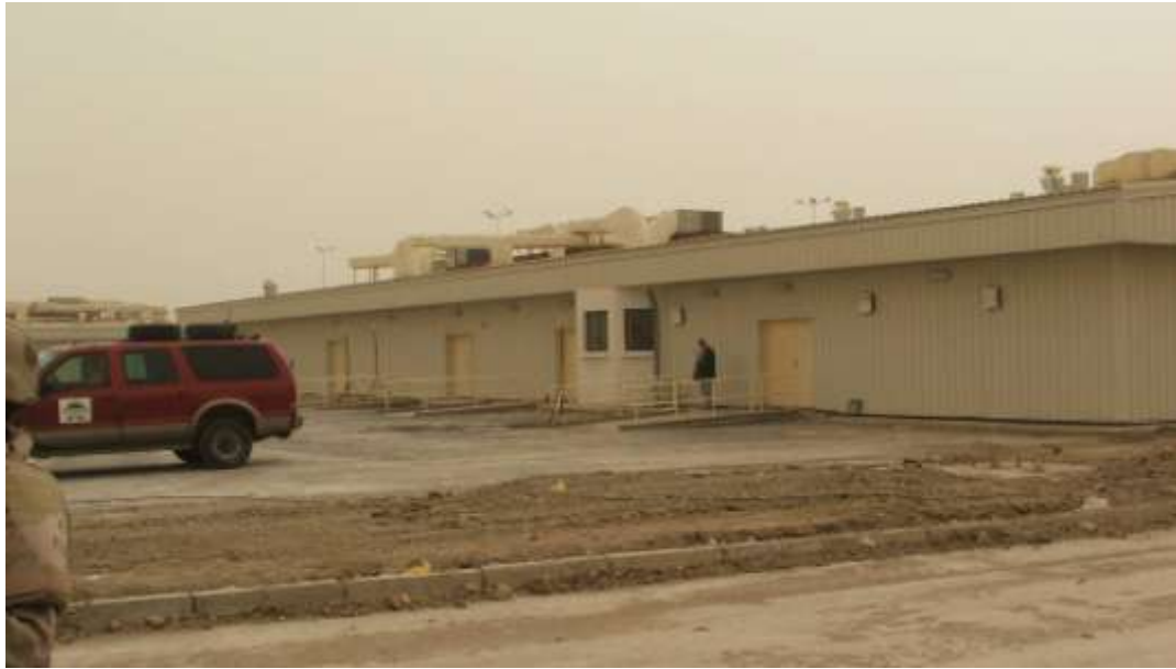
Site Photo 13. Kitchen and laundry building
