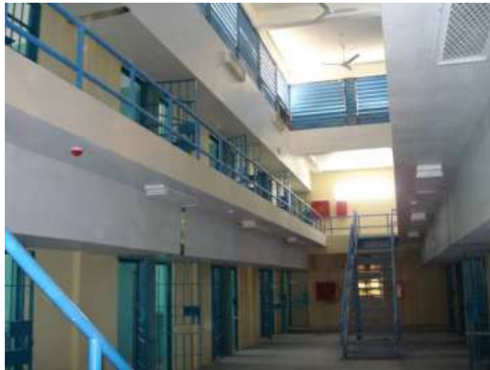
Site Photo 4. Inmate housing corridor one of four (Photo courtesy of the USACE)
