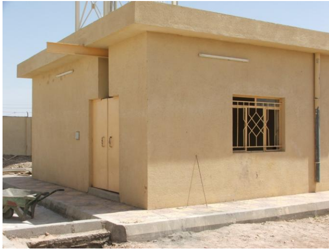
Site Photo 7. Chemical building
