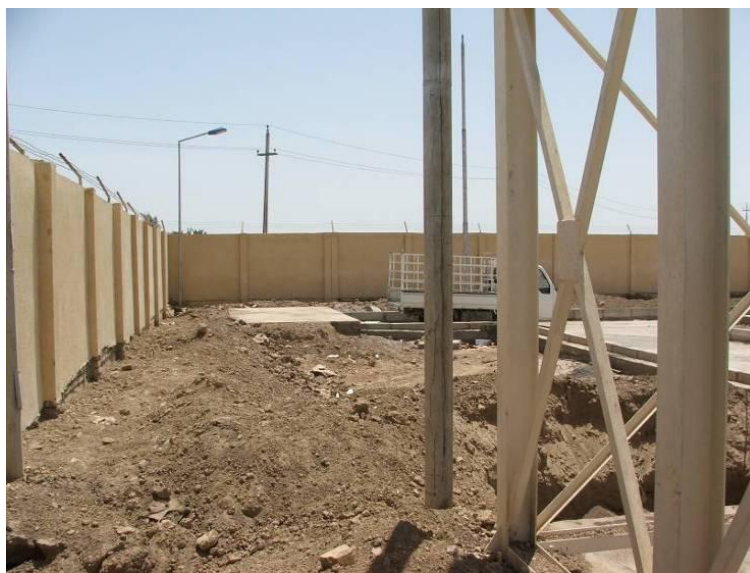
Site Photo 6. Site fencing with barbed wire and perimeter lighting
