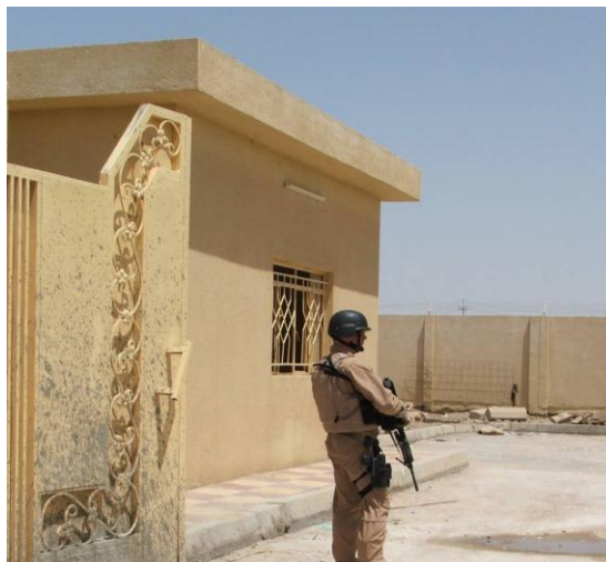
Site Photo 9. Operator building
