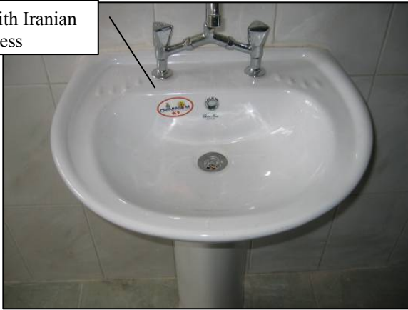
Site Photo 10. Bathroom sink
