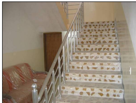
Site Photo 14. Stairway and railing
