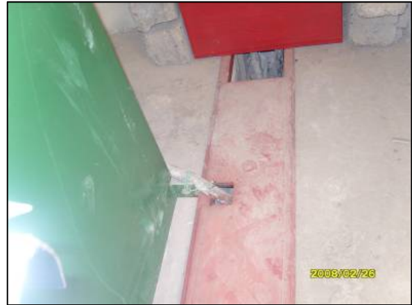
Site Photo 16. Corrective action subsequent to site visit to install automatic turnover box and properly connect to the main line. (Photo courtesy of MND-NE).
