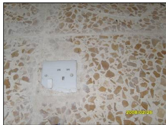
Site Photo 9. Corrective actions subsequent to site visit to recess and cover receptacle. Portion of receptacle obscured. (Photo courtesy of MND-NE).
