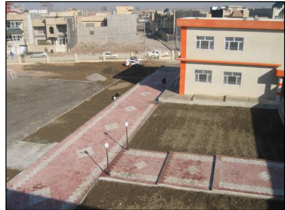
Site Photo 4. Outside building finish
