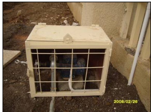
Site Photo 26. Corrective action subsequent to site visit to provide a cover for the pump. (Photo courtesy of MND-NE).
