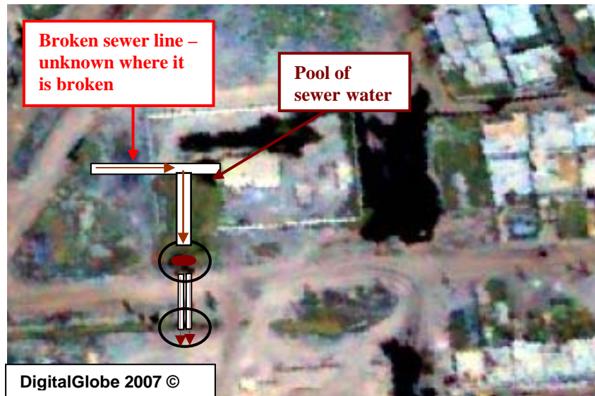
Aerial Image 5. Aerial view of the flow of sewer water from the manhole outside the G-7 lift station to the next available manhole across the street
