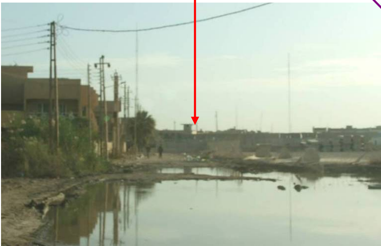
Site Photos 4 and 5. Backed-up sewer water in the Al Ghazaliyah area of Baghdad
