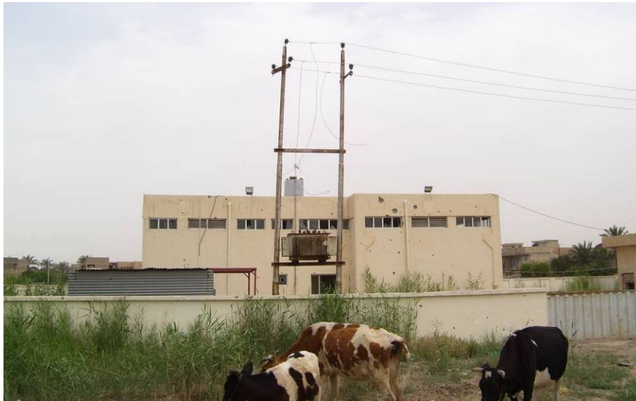
Site Photo 1. Exterior view of the Al Ghazaliyah G-7 Sewage Lift Station
