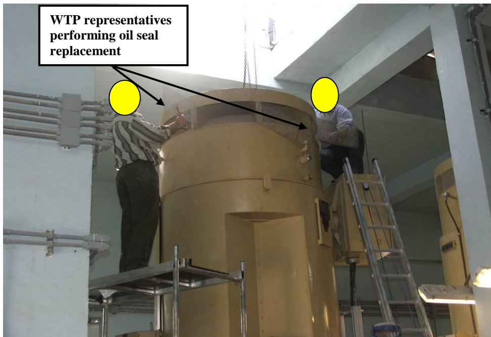
Site Photo 23. A vertical turbine pump being repaired by WTP representatives
