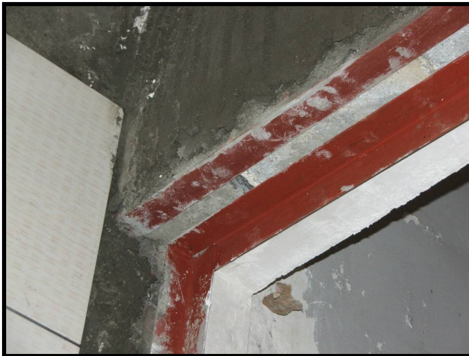
Site Photo 14. Typical steel door frame installation.
