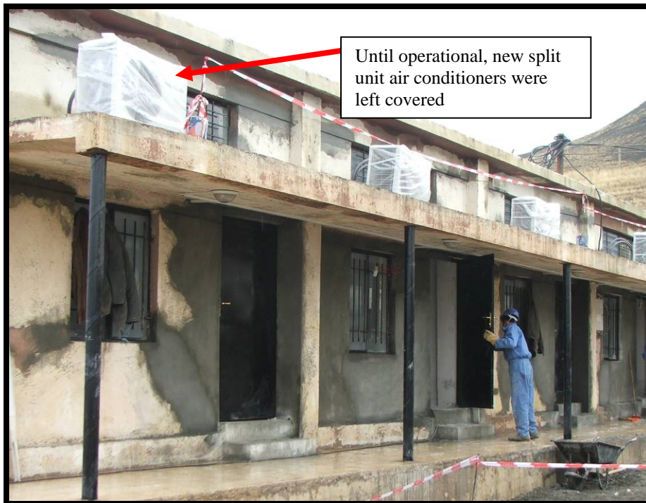
Site Photo 11. Exterior renovation work in progress.
