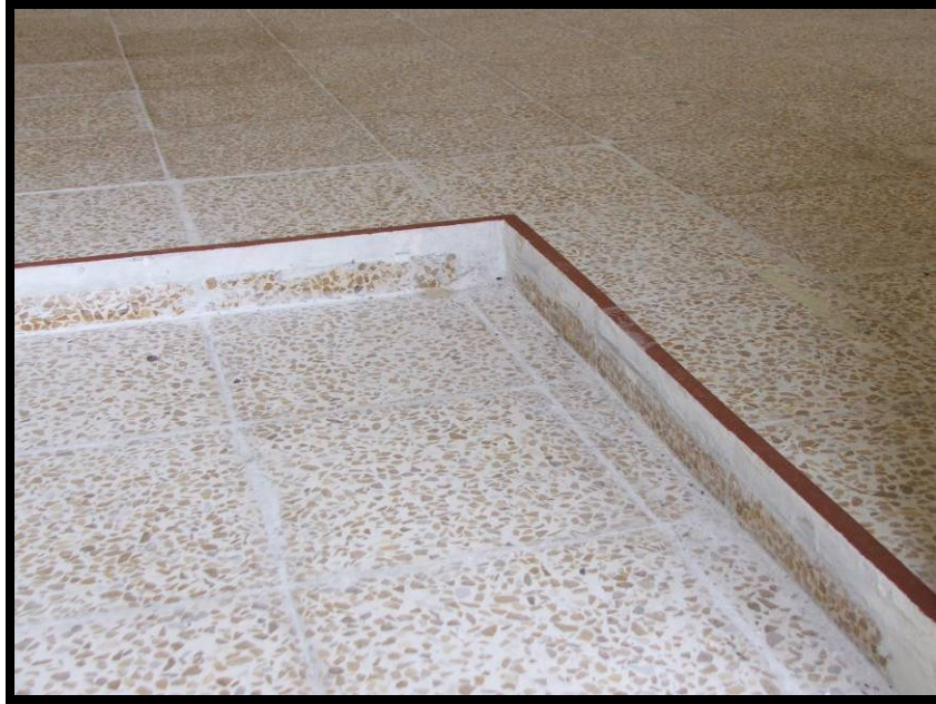
Site Photo 13. New Terrazzo floor included lowered entry area.
