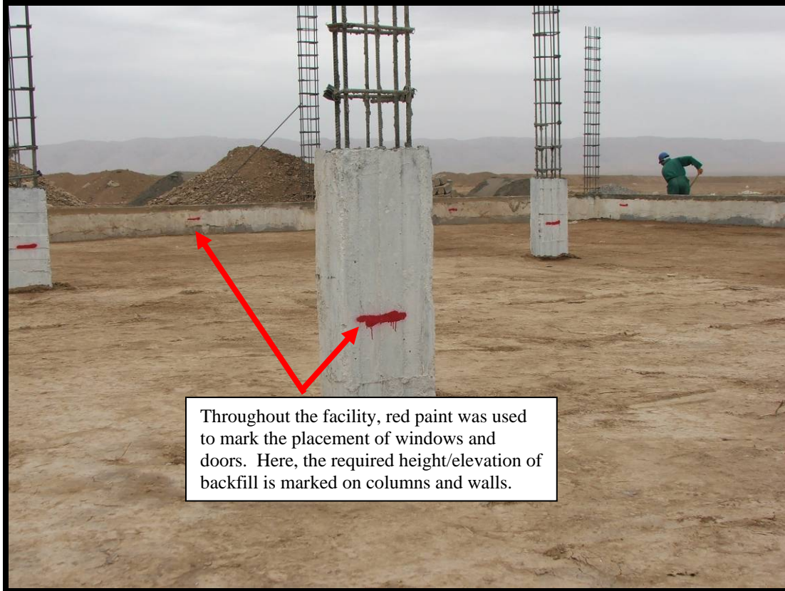
Site Photo 2. Backfill requirement marked.
