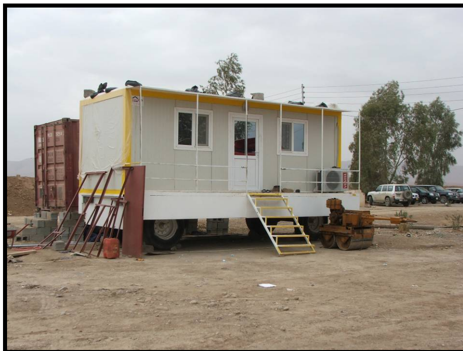
Site Photo 20. Subcontractor construction office.
