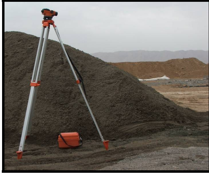
Site Photo 16. Transit was setup and ready when needed.
