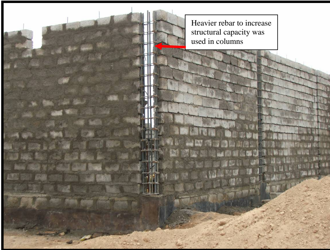
Site Photo 18. Typical wall construction before forming and casting columns.
