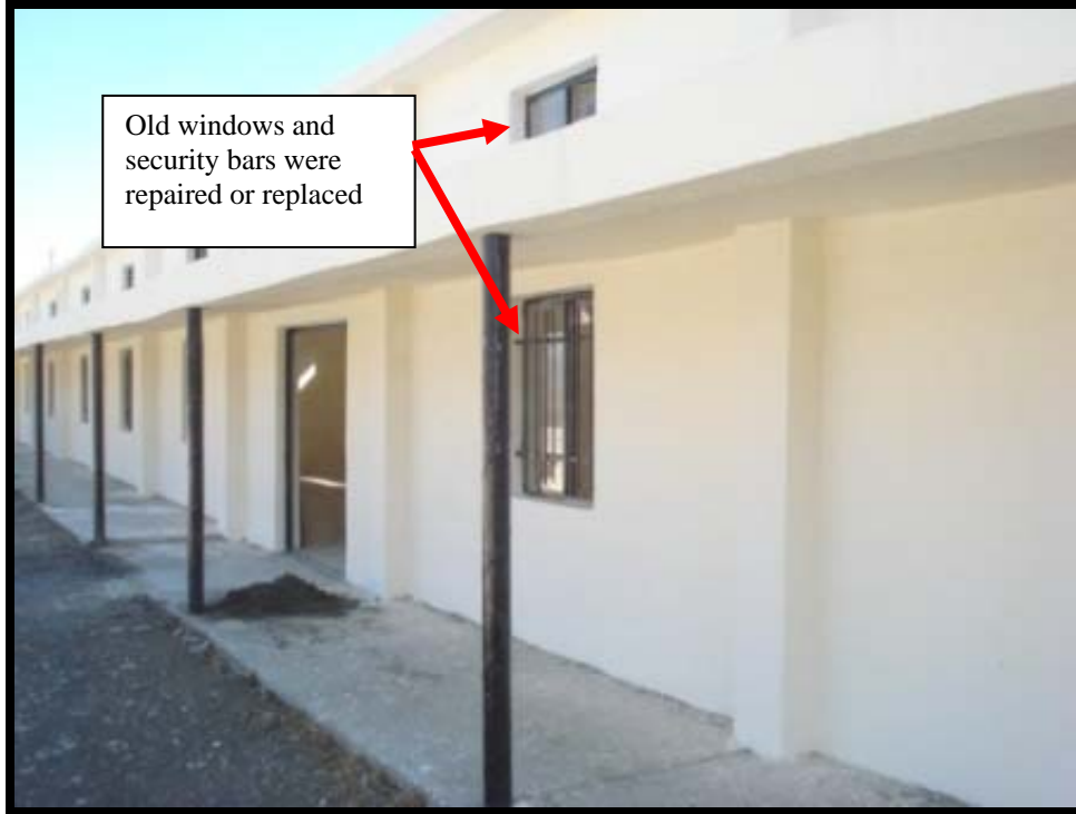
Site Photo 10. Typical building exterior following renovation. (Photo courtesy of Toltest)
