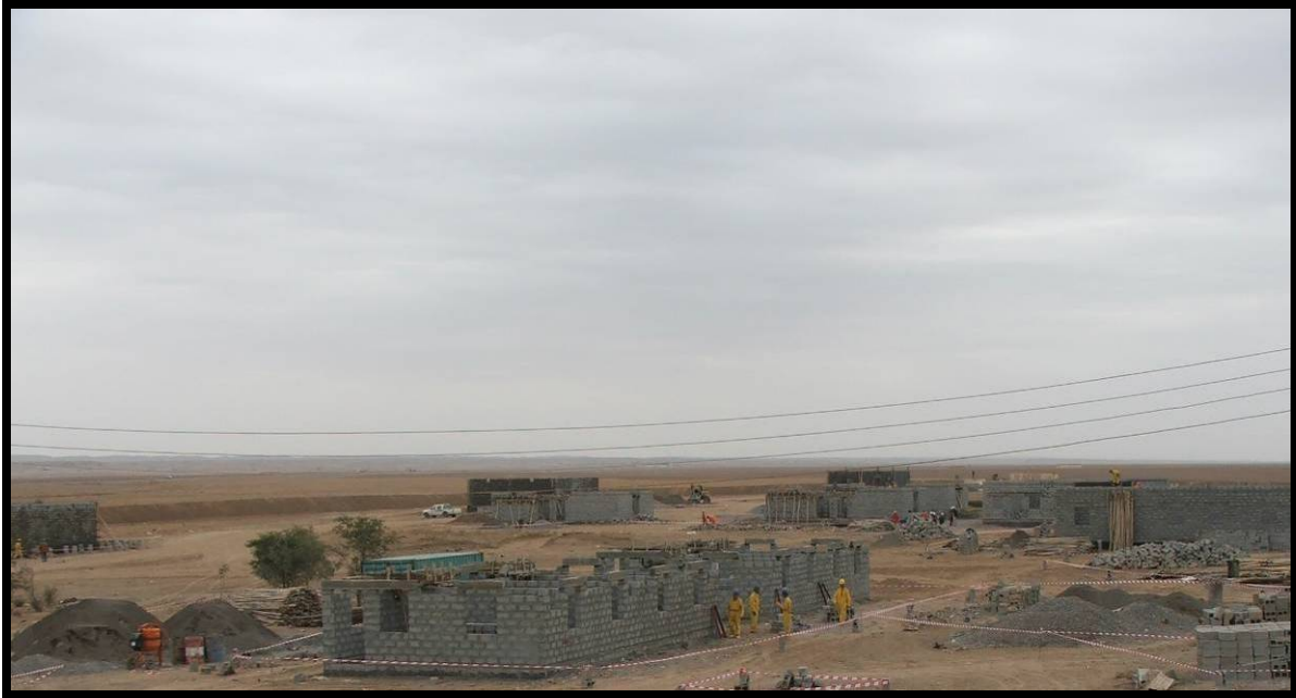
Site Photo 4. Debecha construction activity and flat building site.
