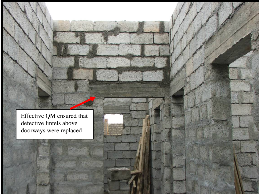
Site Photo 1. Subcontractor reworked lintels.
