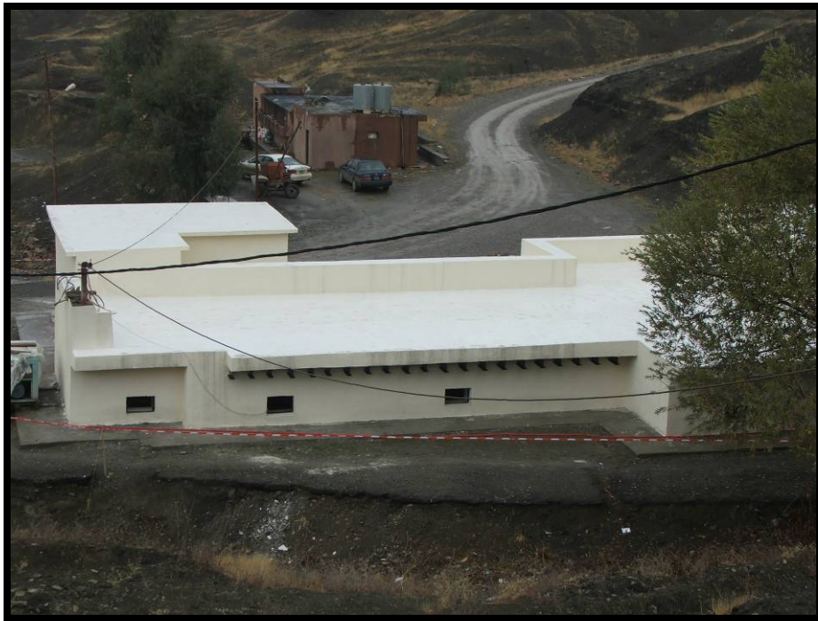
Site Photo 8. Typical roof top following renovation.
