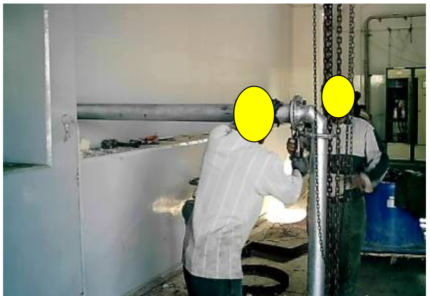
Site Photo 3 and 4. Contractors installing the galvanized pipe for the submersible pump. (Photos courtesy of USACE)
