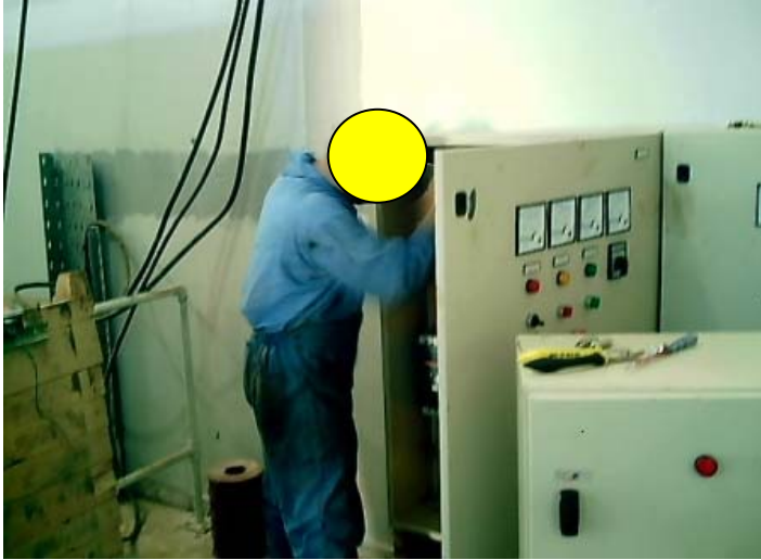
Site Photos 1 and 2. Contractor installation of the electrical control panels and the installed control panels. (Photos courtesy of USACE)
