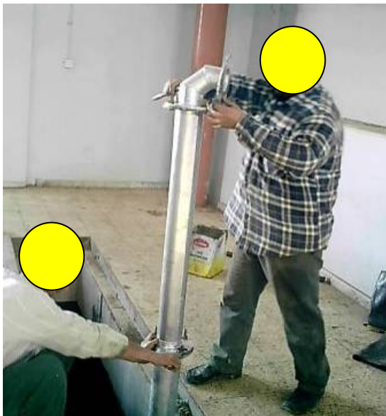
Site Photo 3 and 4. Contractors installing the galvanized pipe for the submersible pump. (Photos courtesy of USACE)
