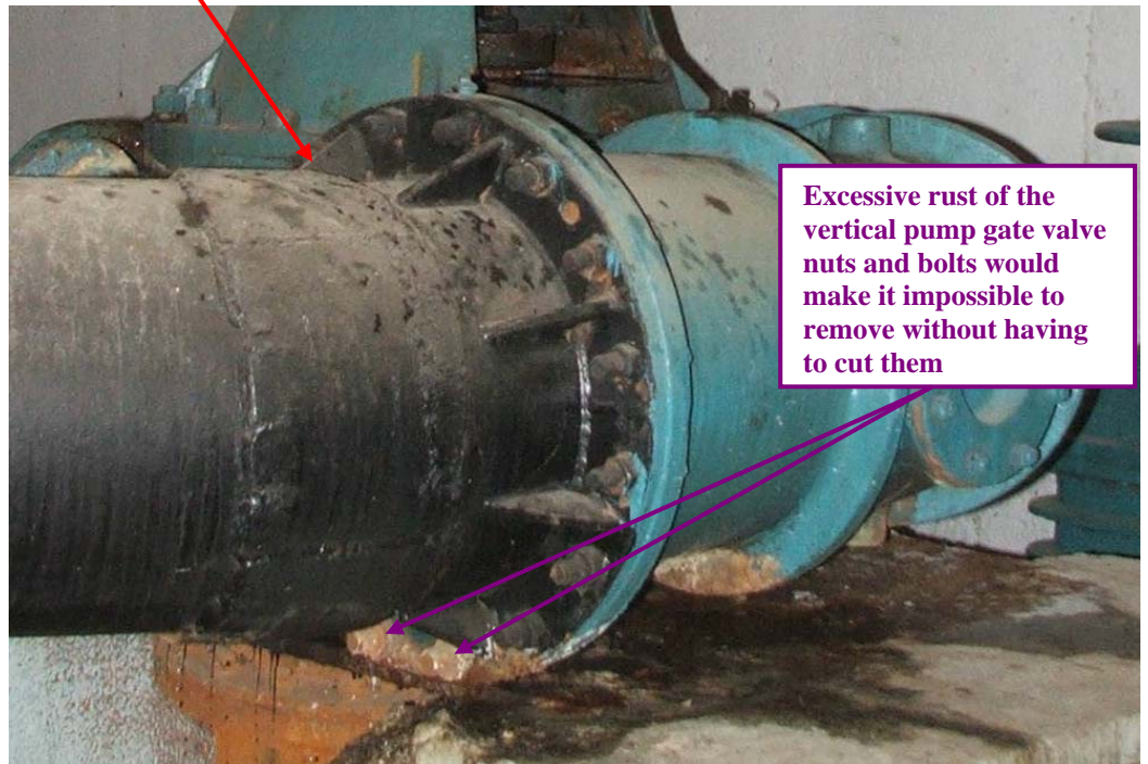
Site Photo 32. Close up view of Site Photo 31
