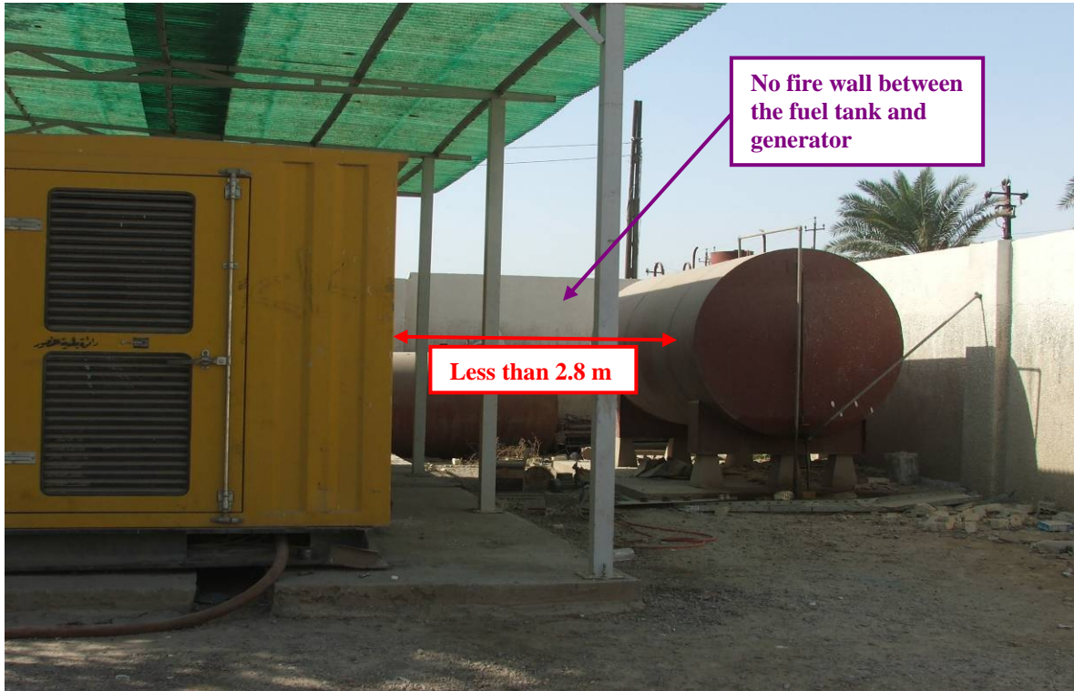
Site Photo 35. Location of the pump station fuel tank
