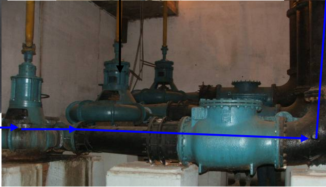
Figure 1. Flow of sewer water into and out of the Mansour Pump Station in the Al Amerea area. Steps 1 through 3 of the pumping process.
