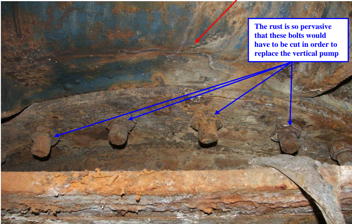
Site Photo 24. Close up view of Site Photo 23
