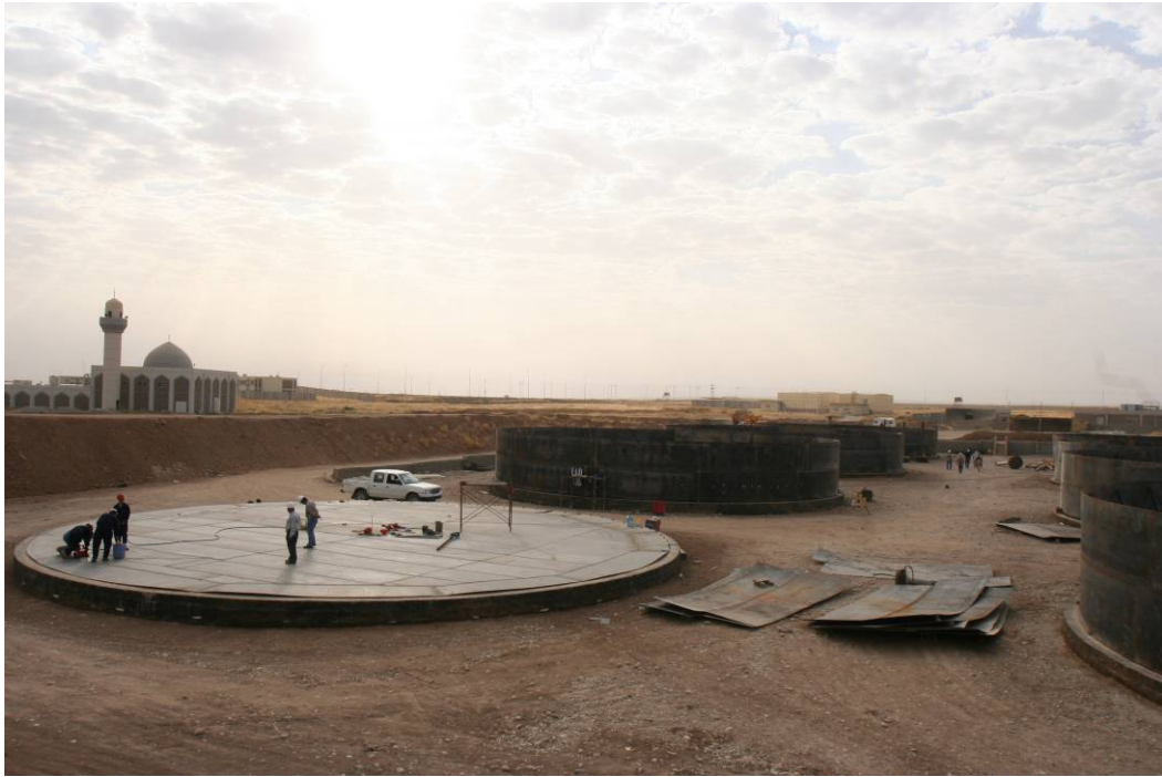
Site Photo 3. Steel floor placed on concrete foundation.
