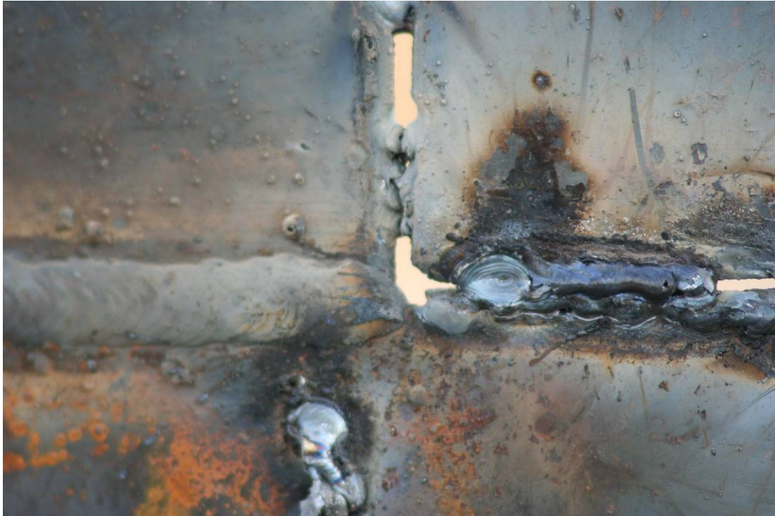
Site Photo 14. Tack welds temporarily attach wall plates together.
