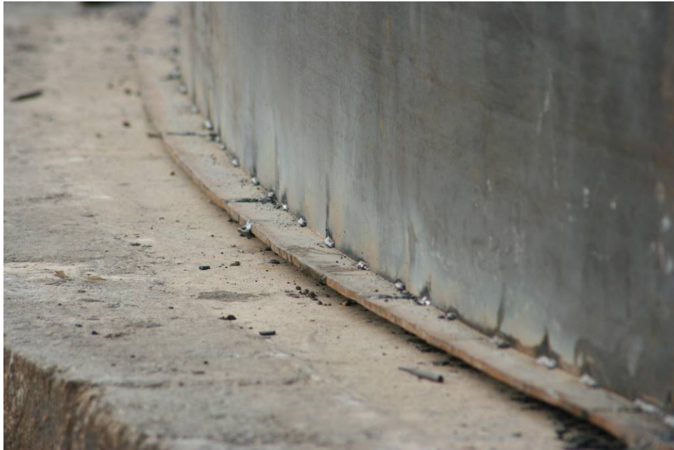
Site Photo 13. Tack welds temporarily attach wall plate to floor.
