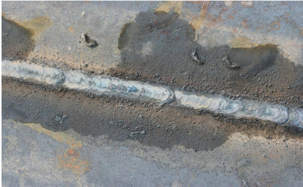
Site Photo 9. High quality annular plate weld.
