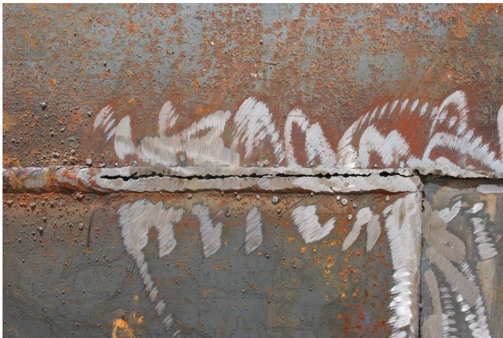
Site Photo 21. Close-up of bead ground flush with plate steel.
