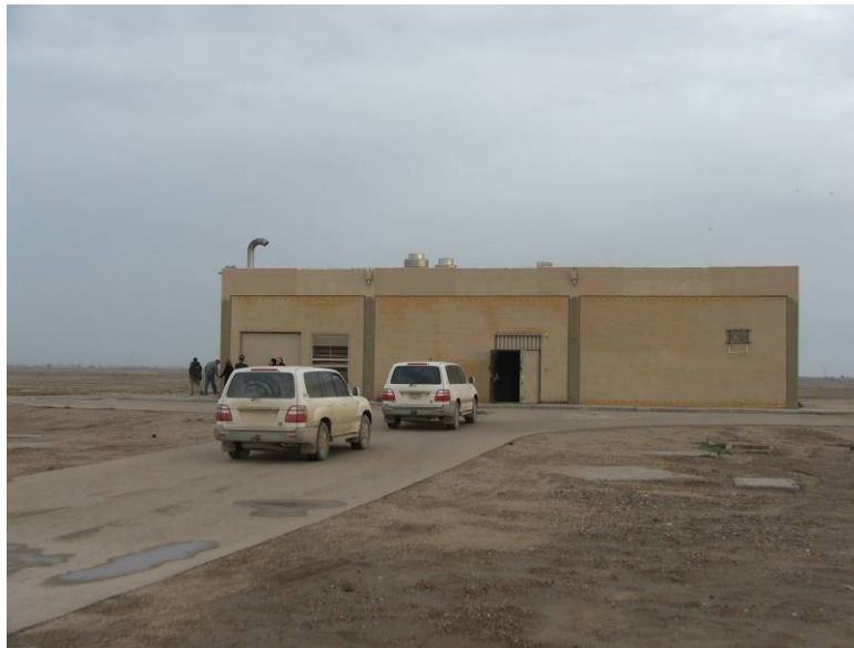
Site Photo 3: Exterior view of S-330 substation
