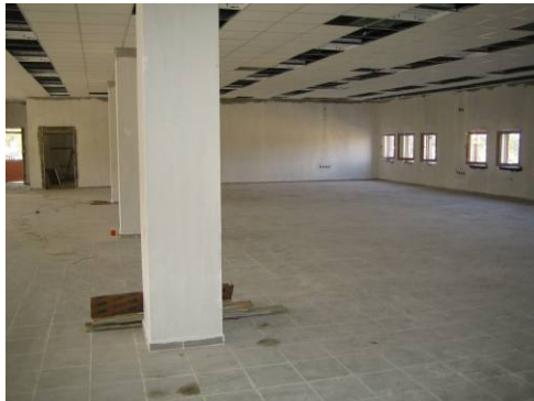
Site Photo 9. Administrative space under construction – Photo provided by MNSTC-I
