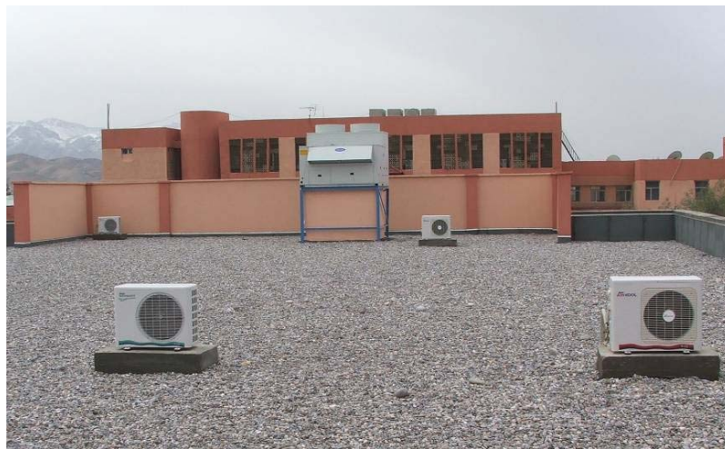
Site Photo 11. Headquarters building roof with roof-top HVAC units
