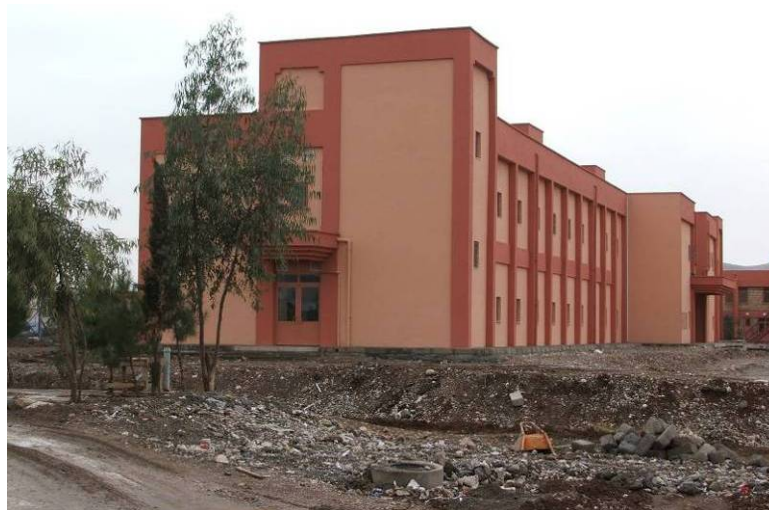
Site Photo 8. Exterior of new barracks facility
