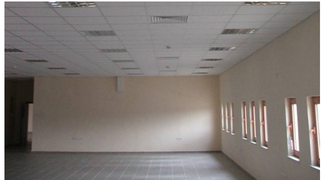
Site Photo 10. Completed administrative space
