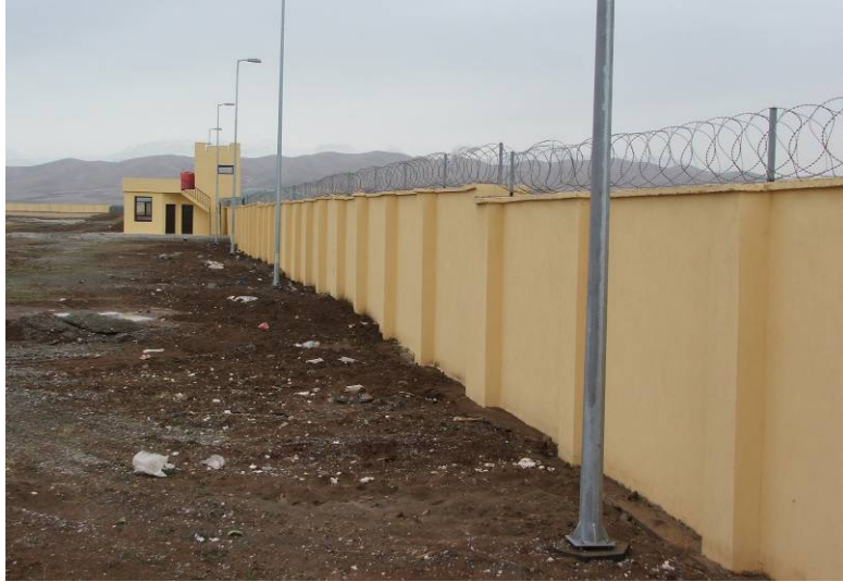
Site Photo 13. The perimeter wall along the north part of the Military Academy
