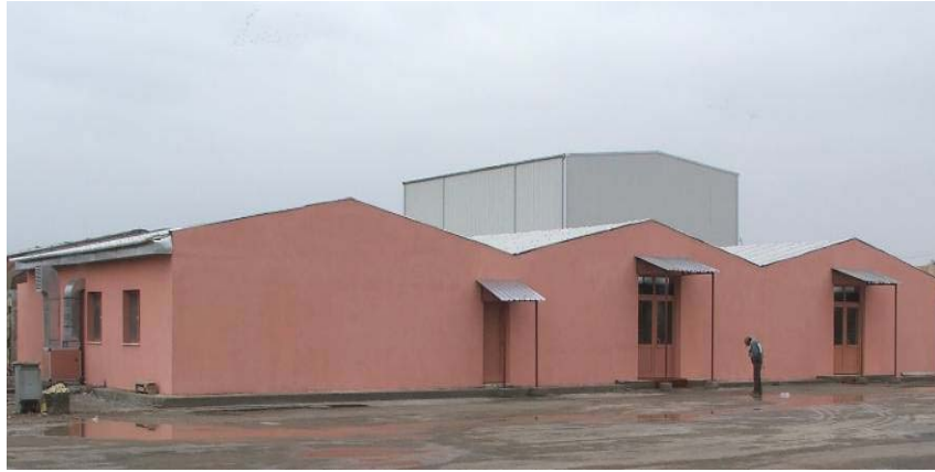
Site Photo 3. Exterior of renovated dining facility (Bldg. 1060)
