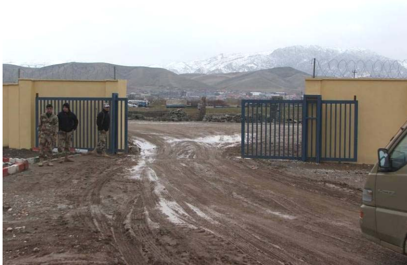
Site Photo 14. Sliding gate along the east wall of the military academy
