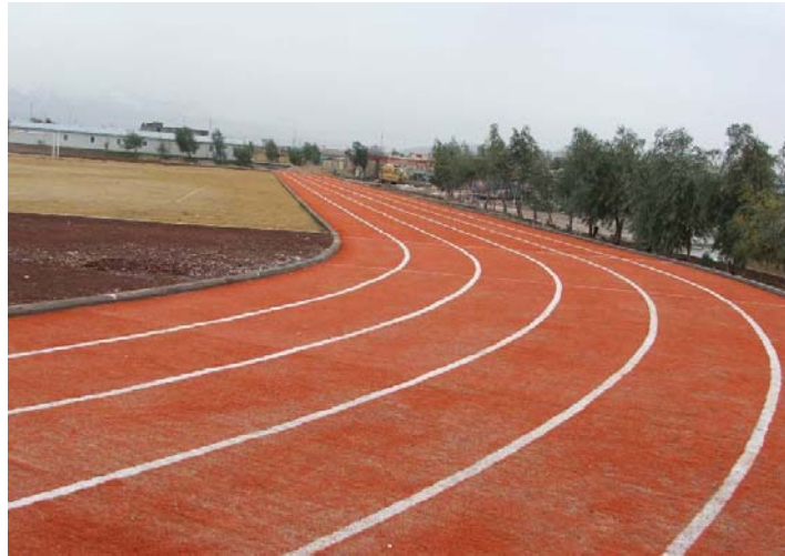
Site Photo 19. Synthetic track surface on the outside of the soccer field
