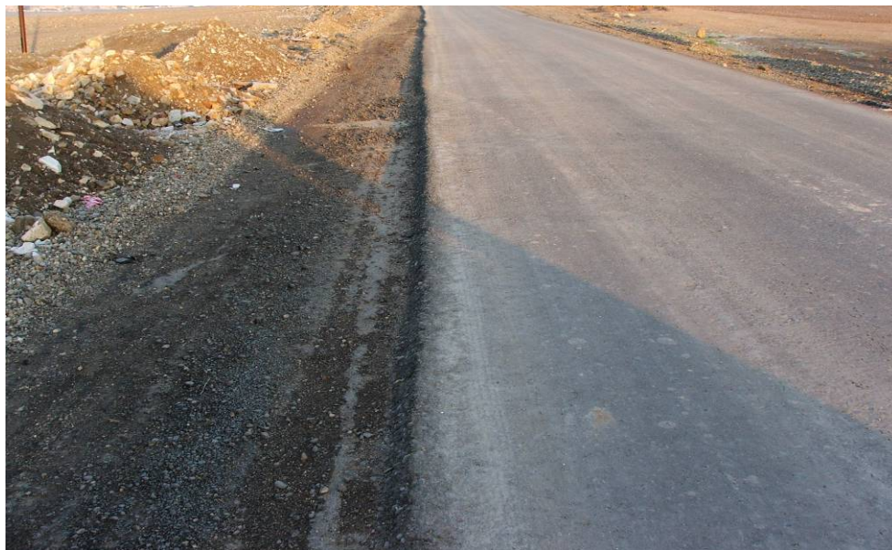
Site Photo 9. Compacted shoulder sub-base
