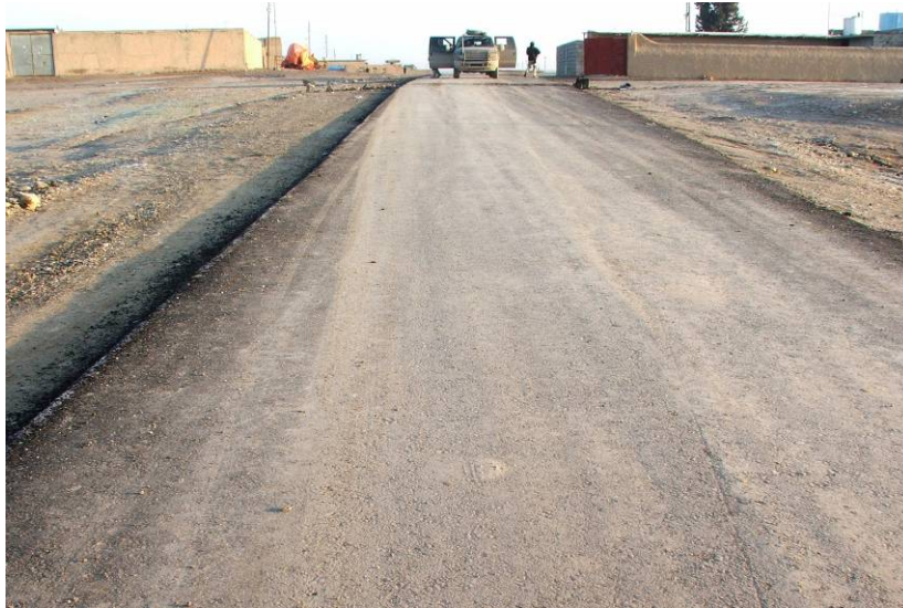
Site Photo 5. Asphalt concrete pavement near village of Balawat
