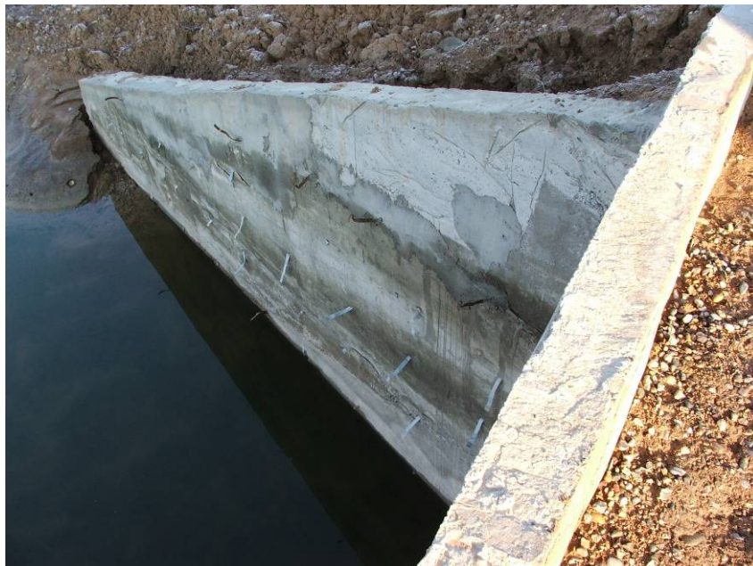
Site Photo 11: Box culvert wing wall
