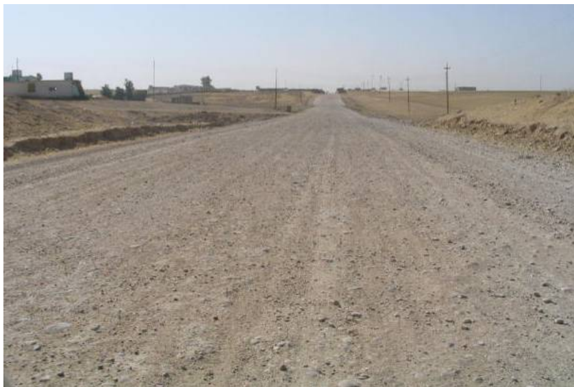
Site Photo 3. Cut section near Balawat – Photo provided by USACE
