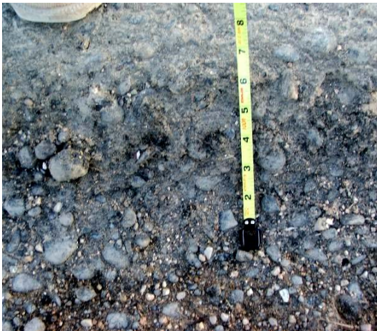
Site Photo 6. Depth of the asphalt base course
