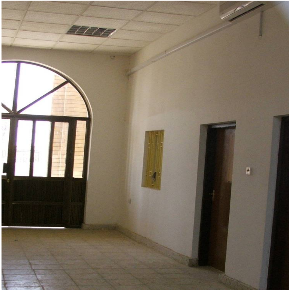
Site Photo 8. Terrazzo Floor Tile Located in the Center Entry Room
