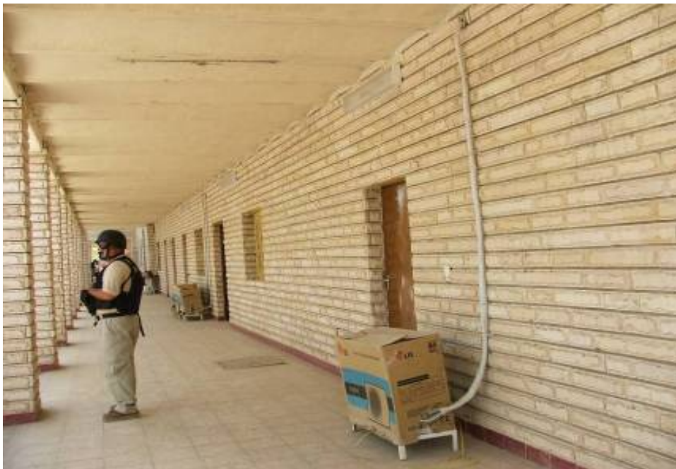
Site Photo 1. Facing Brick on Rear Wall and Columns
