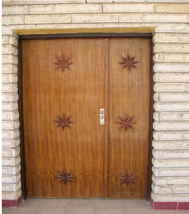
Site Photo 6. Exterior Wooden Door
