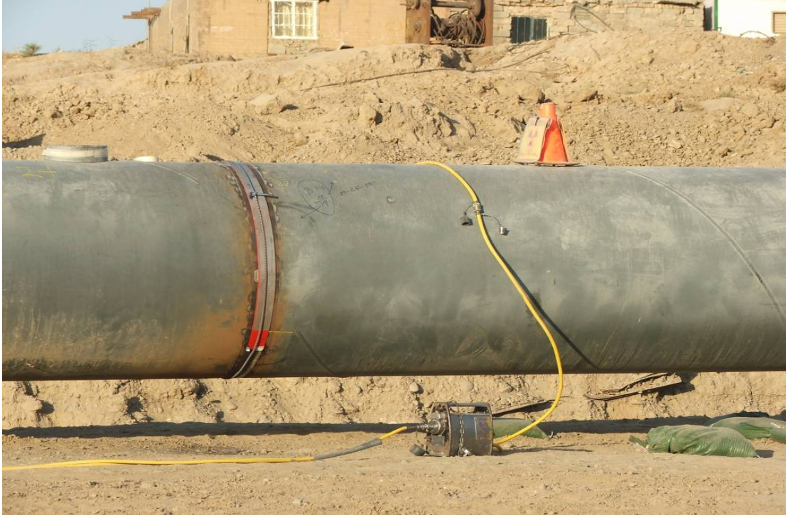
Site Photo 8: Radiography (x-ray) Test In Progress on 40-inch Pipe Weld
