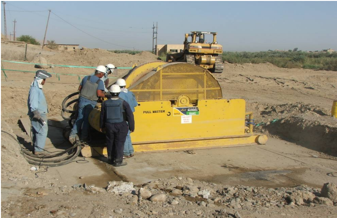
Site Photo 13: Field Supervisor Oversees Winch Cable Change-Out
