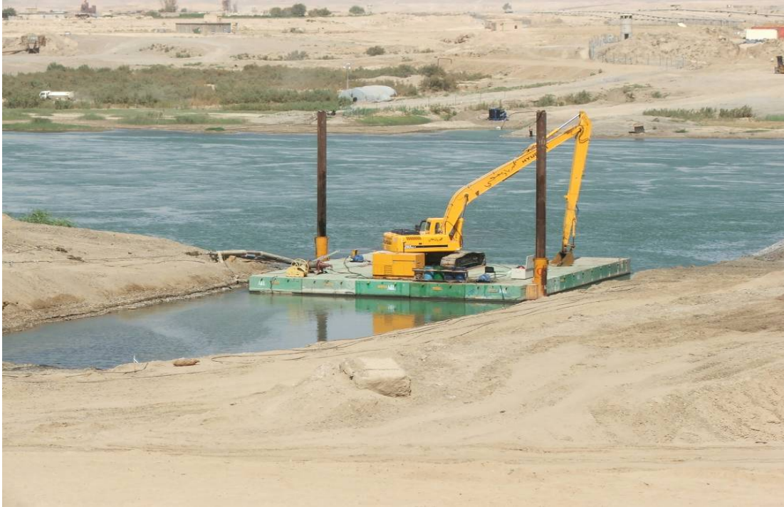
Site Photo 5: Excavator for Dredging on Tigris River
