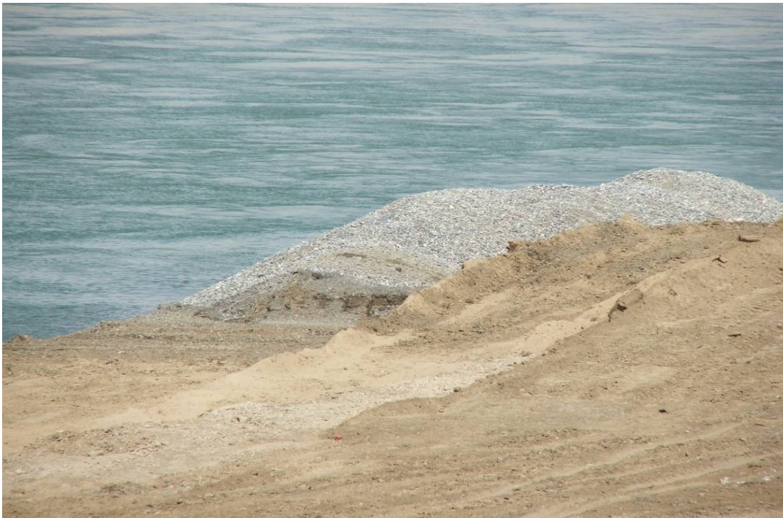
Site Photo 4: River Rock and Gravel Dredged from River Bed
