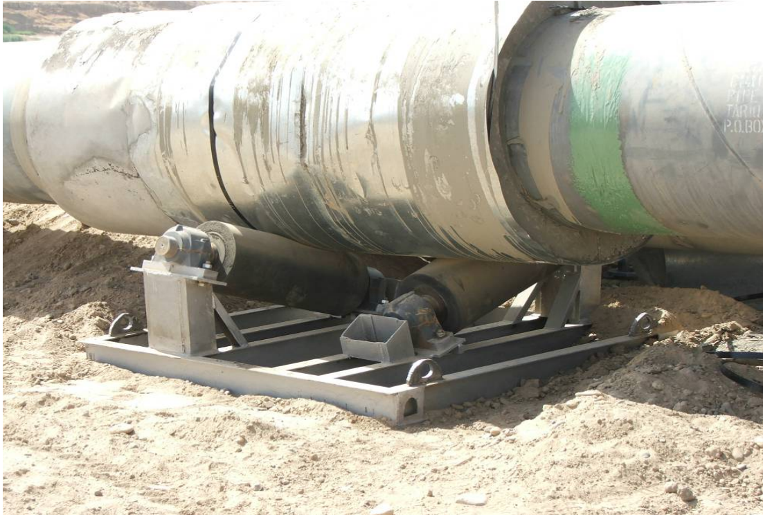
Site Photo 1: 40-Inch Pipeline on Rollers
