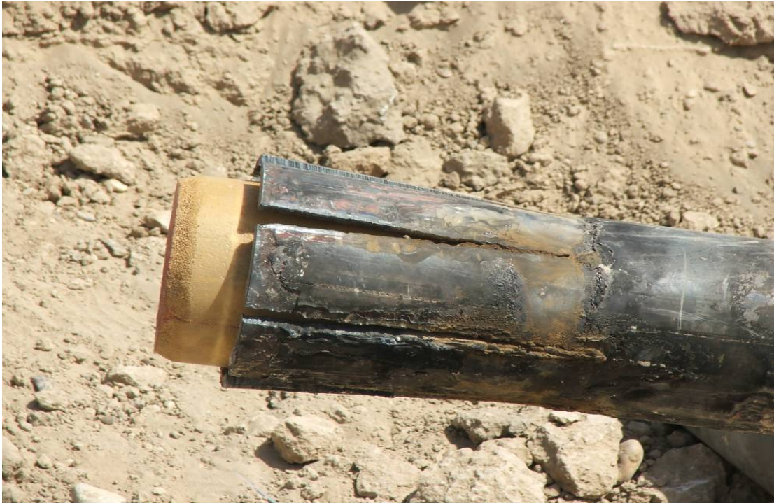
Site Photo 7: Pipe Ready for Pigging
