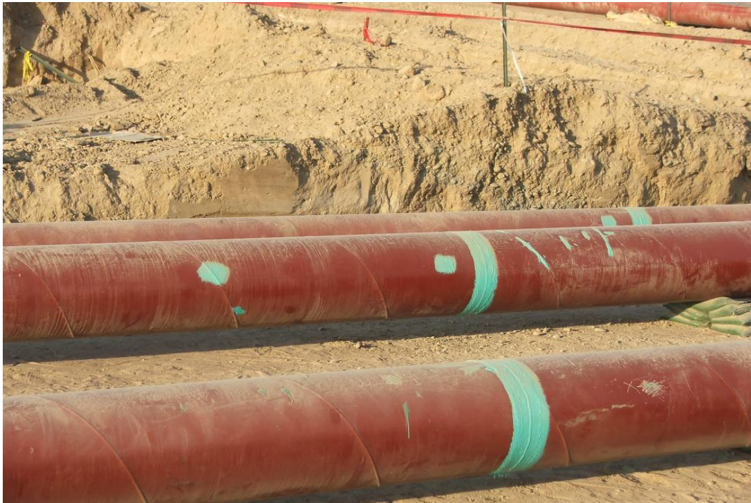
Site Photo 9: Corrosion Control Epoxy Following Holiday Test
