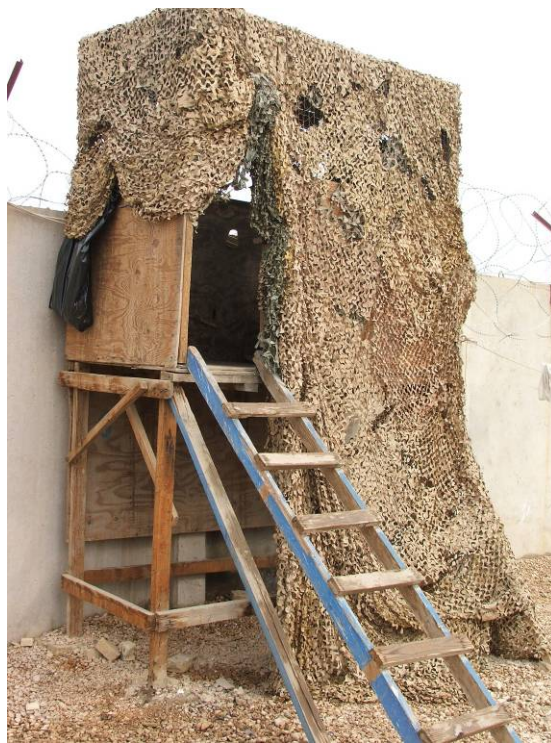
Site Photo 14. Guard Tower at the Hillah Police Academy
