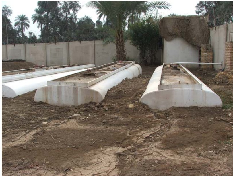
Site Photo 13. Wastewater Collection Tanks Partially Buried
