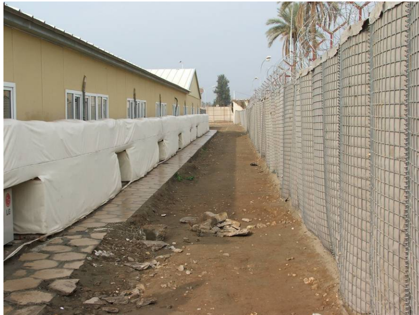
Site Photo 11. Hesco Wall Reinforcing the Outside Concrete Perimeter Wall
