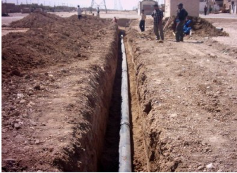
Photo 2: Installation of 200 mm UPVC pipeline
