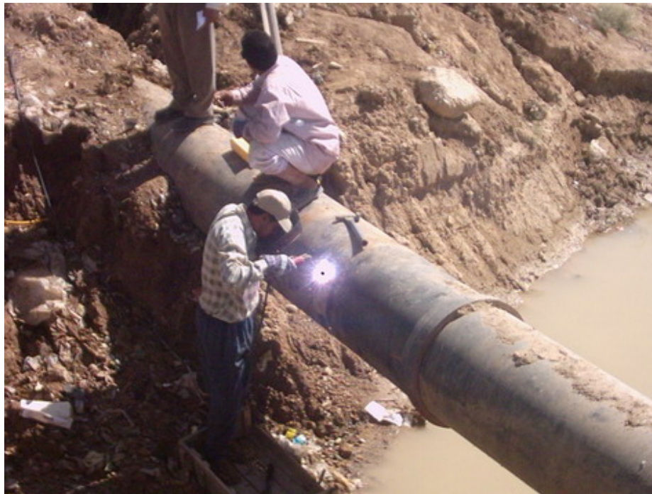
Photo 7: Repair of water main after disconnecting illegal connection
