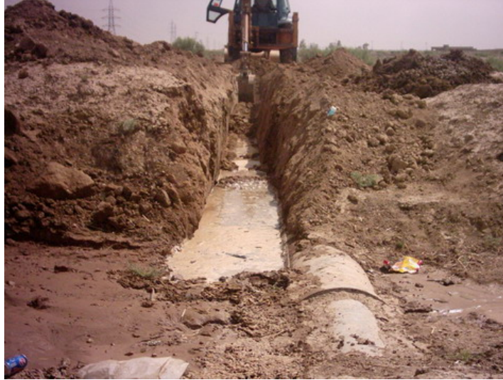
Photo 4: Excavation to locate illegal connections
