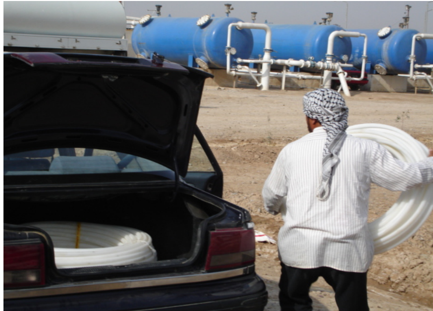
Photo 8: Arrival of 15 millimeter water line used for house connections
