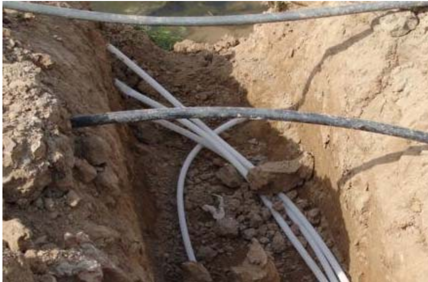
Photo 9: Placement of 15 millimeter water lines in excavation
