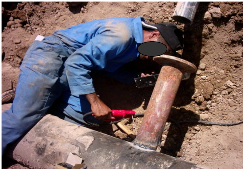
Photo 1: Installation of connecting flange to the 450 mm water main
