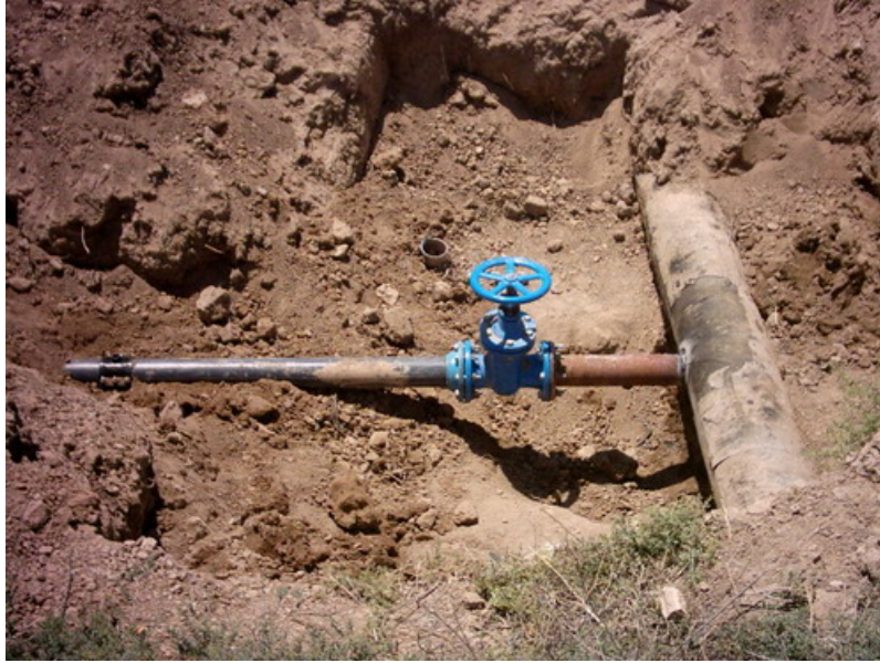
Photo 3: 110 mm connection to 300 mm existing pipe
