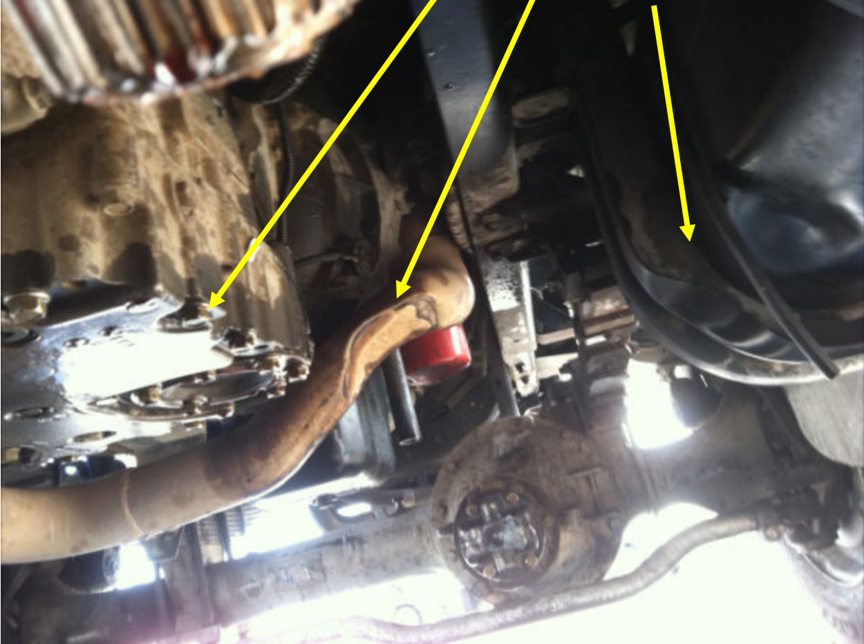
Figure 7 View from transfer case (note damage to transmission, exhaust, and fuel tank)
