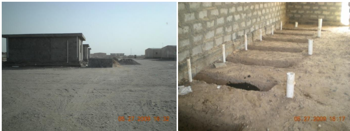
Figure 4—Example of the exterior and interior construction status of latrines
