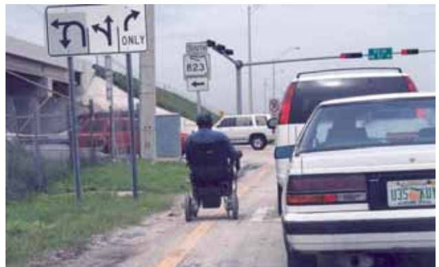
Figure 39. Missing Sidewalk Links and Lack of Facilities for Pedestrians.
