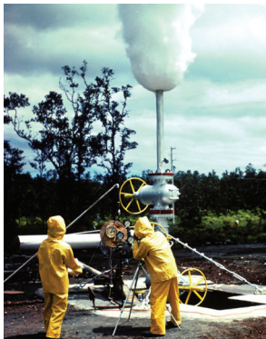
Left: Pressure testing in 1976 of a geothermal well drilled into Kīlauea's lower east rift zone. A power plant later constructed in this area produces about 30 megawatts of electricity, about 30 percent of the island's needs. (Photograph courtesy of the Hawai'i Geothermal Project.) Right: Some of the power-generating equipment at this plant, the only commercial producer of geothermal energy in the State of Hawai'i. (Photograph courtesy of Puna Geothermal Venture.)
