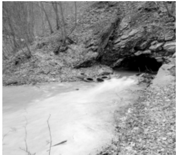
This mine opening, or entry portal, in Eastern Pennsylvania was abandoned in the early 1900's. Today, a large quantity of acid mine drainage flows from the open portal polluting rivers many miles downstream.
