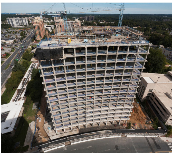
New NRC Headquarters Building Construction Site
