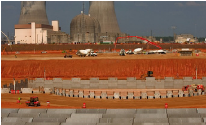
Vogtle New Reactor Site
