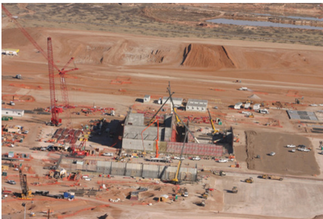
Construction at the URENCO Enrichment Facility
