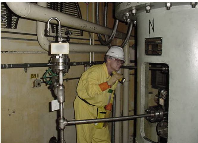
NRC Employee Conducting an Inspection at Byron Nuclear Plant
