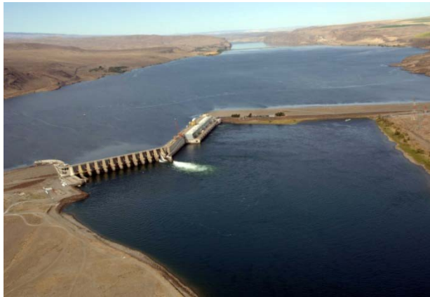
Figure 8-7. Large hydroelectric plant
