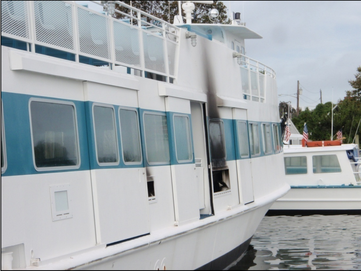
Figure 4. Soot damage to vent opening on starboard side of vessel.
