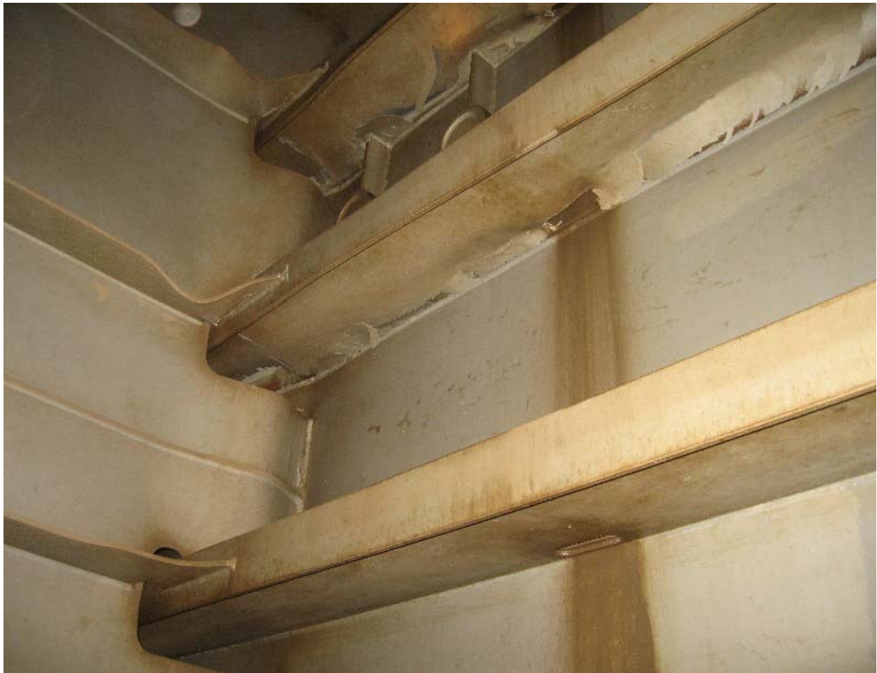
Figure 6. Photo of damage to the interior hull, showing deformation and cracks in the starboard side longitudinals.
