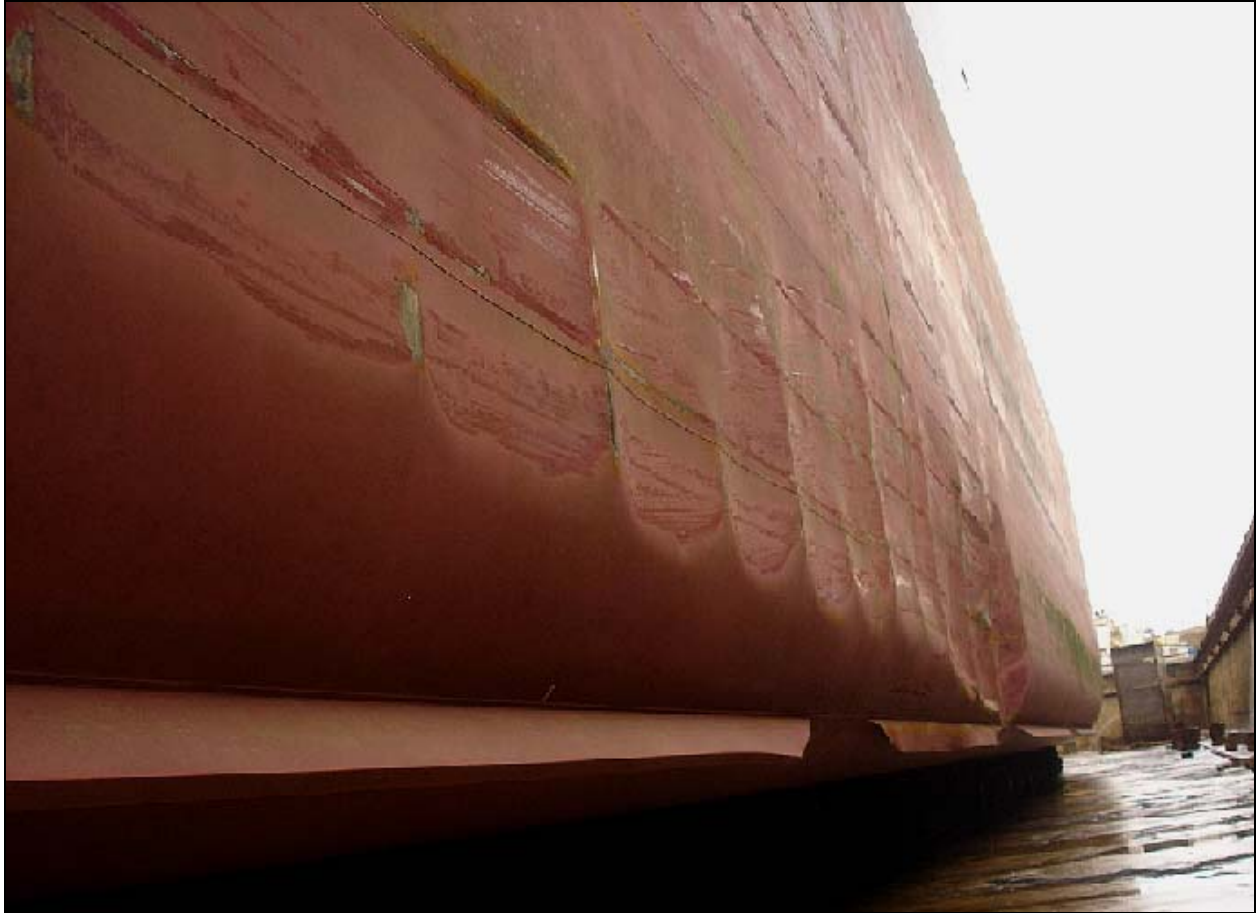
Figure 7. Photo of damage to the exterior starboard hull, showing buckled, scraped steel plates.
