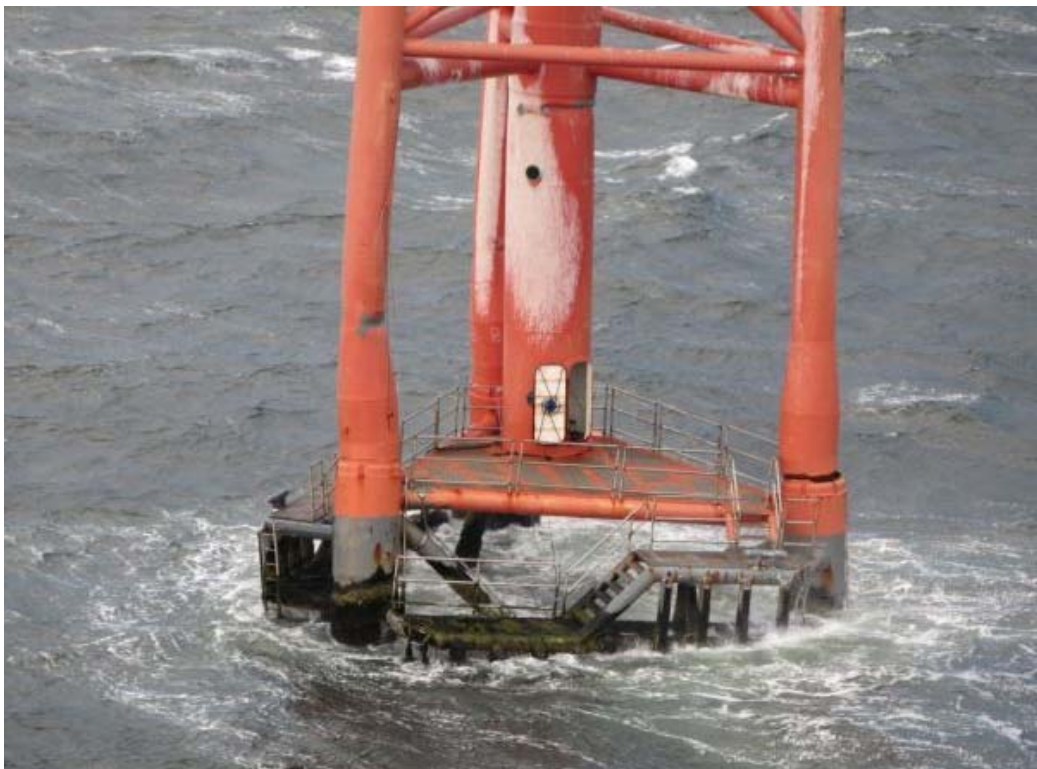
Figure 9. Damage to Ambrose Light. Photo by the Coast Guard.
