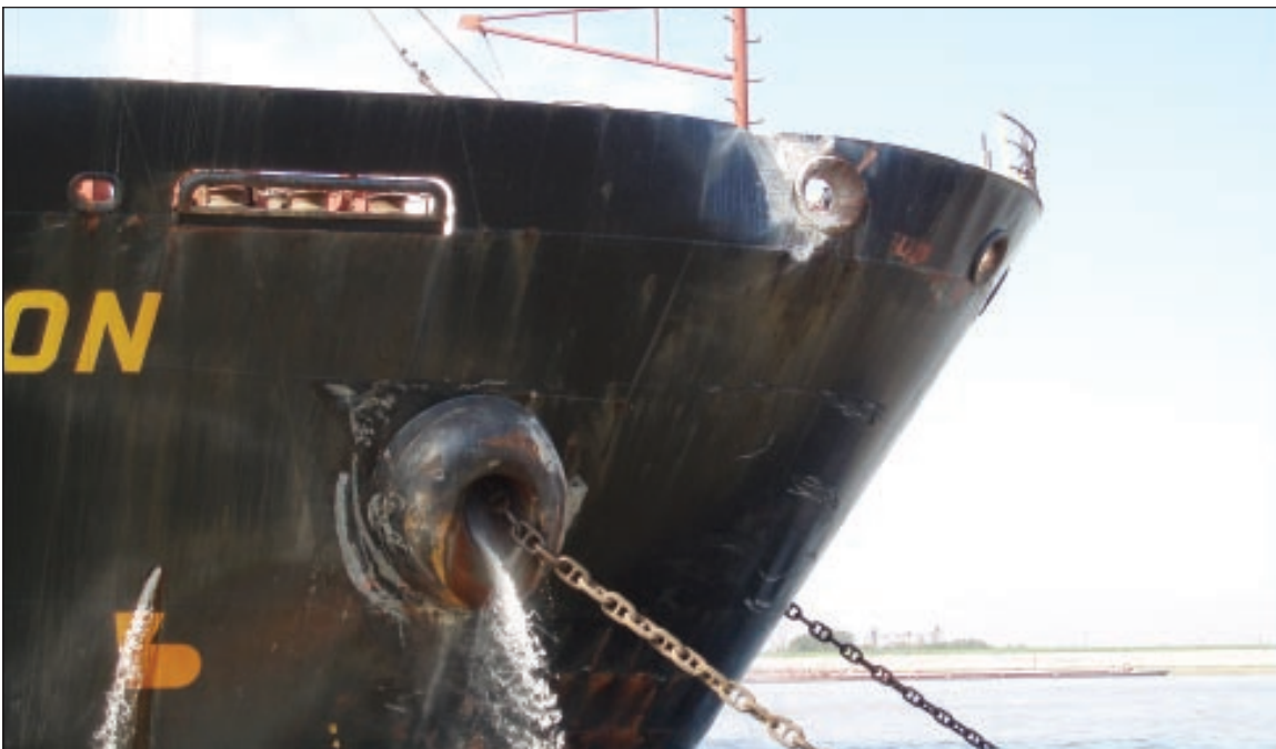
Figure 4. Damage to the bulwark on the Kition's starboard bow.
