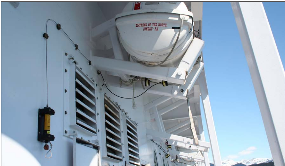
Figure 6. Liferaft remote-release unit mounted on a bulkhead near one of the liferafts.
