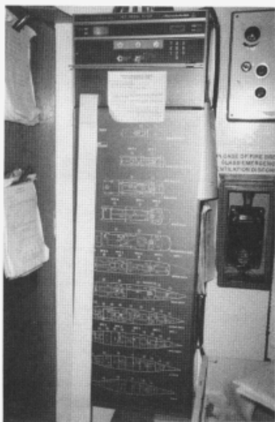
Figure 3—(Left) The fire alarm panel on the bridge showed a plan view of each deck. When an “addressable” fire detector was triggered, a corresponding panel light turned on, indicating the location of the detector. The panel generated a paper log of all activated fire detectors. The tape shown (left of the deck plans) is of the alarms logged during the Universe Explorer fire. (Right) Table shows order of alarms.
