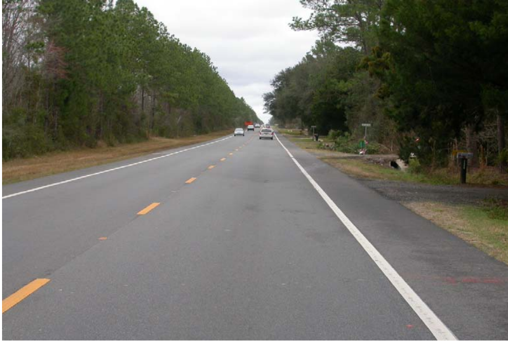
Figure 2. SR 121 approaching accident location.
