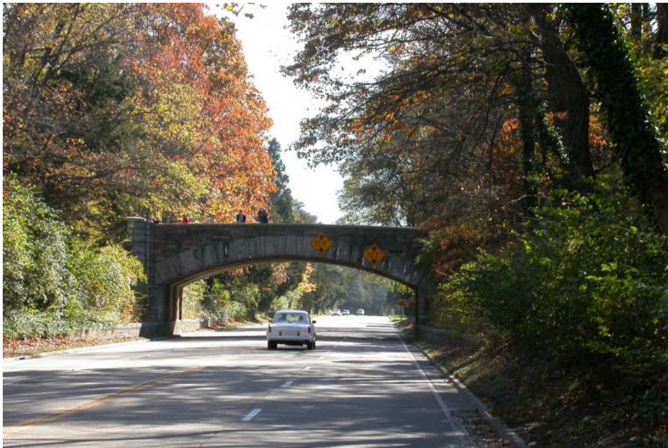
Figure 2. Alexandria Avenue bridge over the Parkway (southbound).
