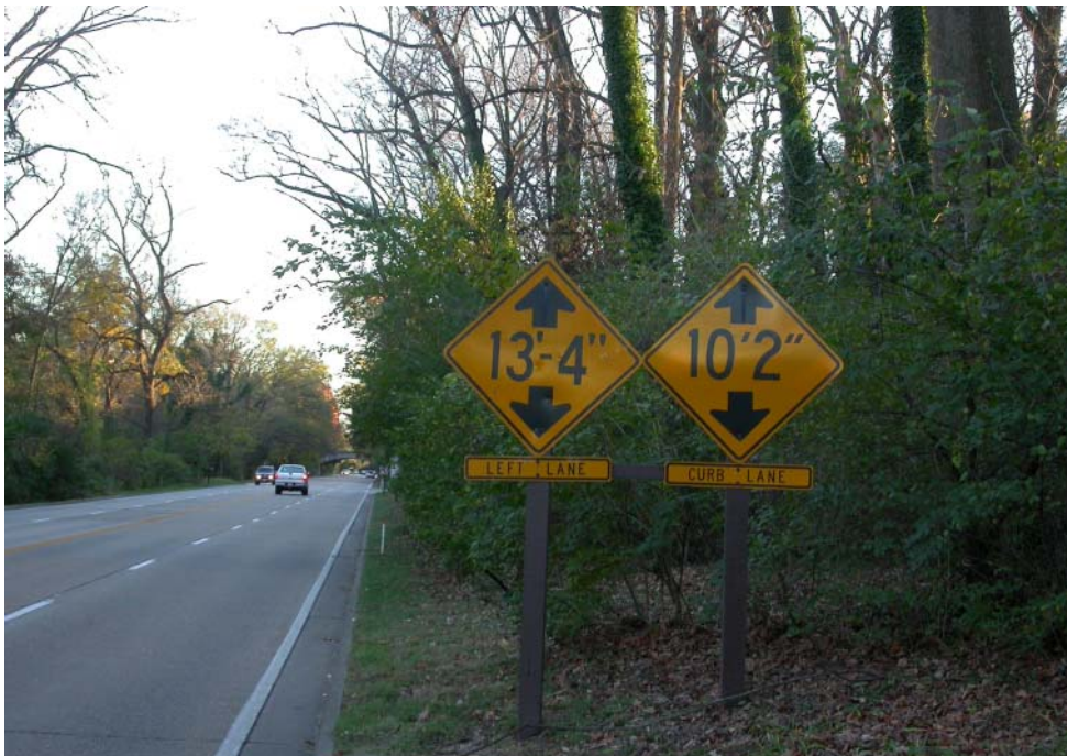
Figure 3. Roadside warning signs—Alexandria Avenue bridge clearance.
