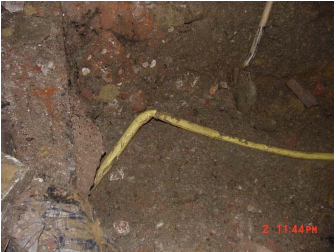
Figure 1. Pulled natural gas service line.
