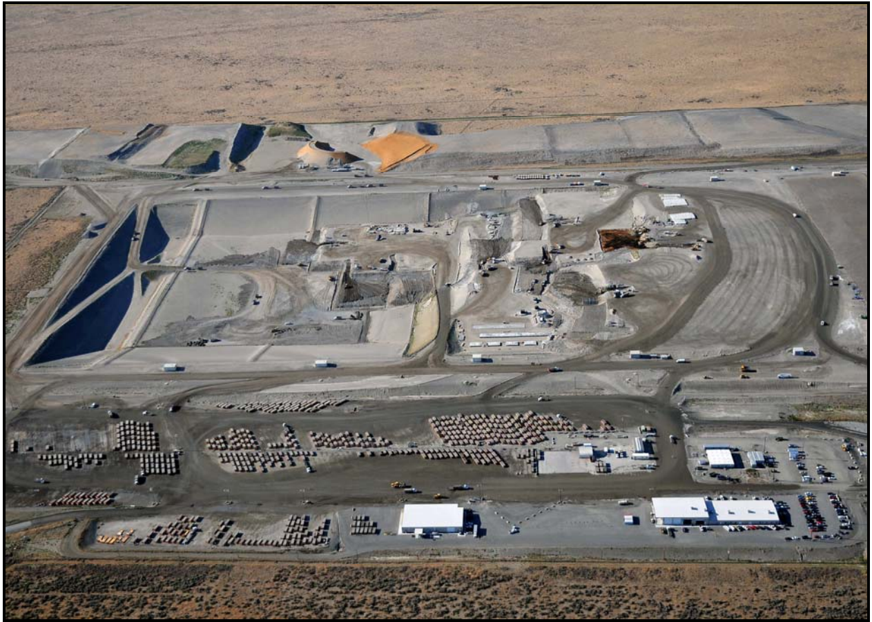
An aerial view of the Environmental Restoration Disposal Facility from the north shows waste being disposed in super cells 9 and 10, left. (Photo 1)
